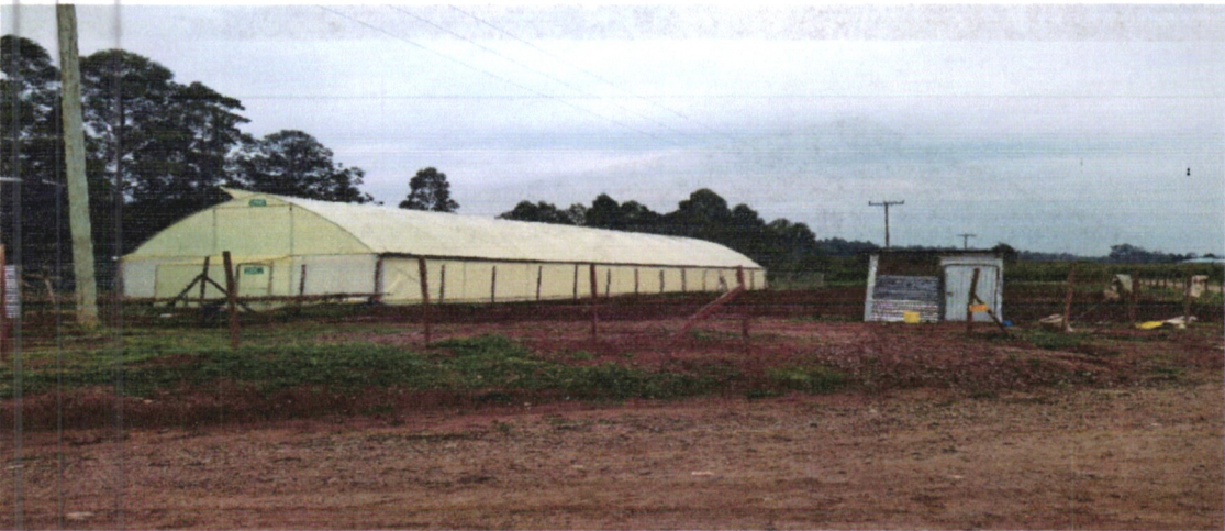
Green House for EPIVOT Project , A partnership between Siala TTI and Meru University.(Above)
