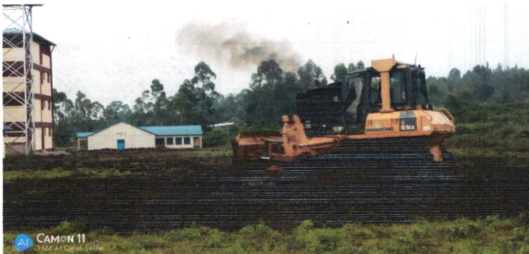
Preparation of the drainage system and rehabilitation of water ways below.
