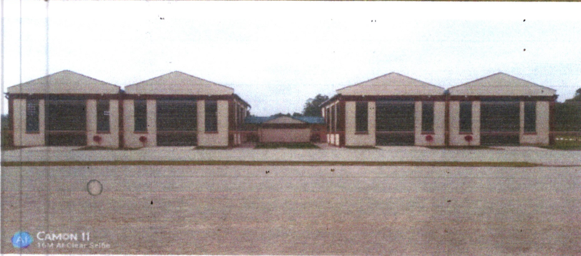
Civil engineering complex above.
