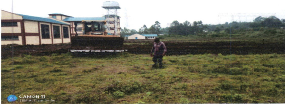
Drainage system preparation above.
