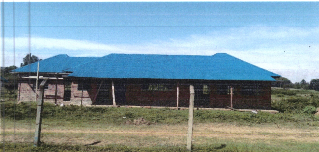
TOP.tuition block under construction
