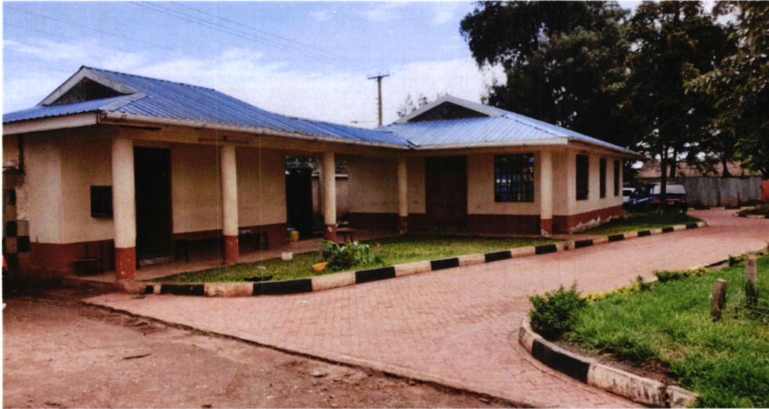
Photo 16: CWSK Nanyuki TPS Health Centre, Reception & Guard house Complete
