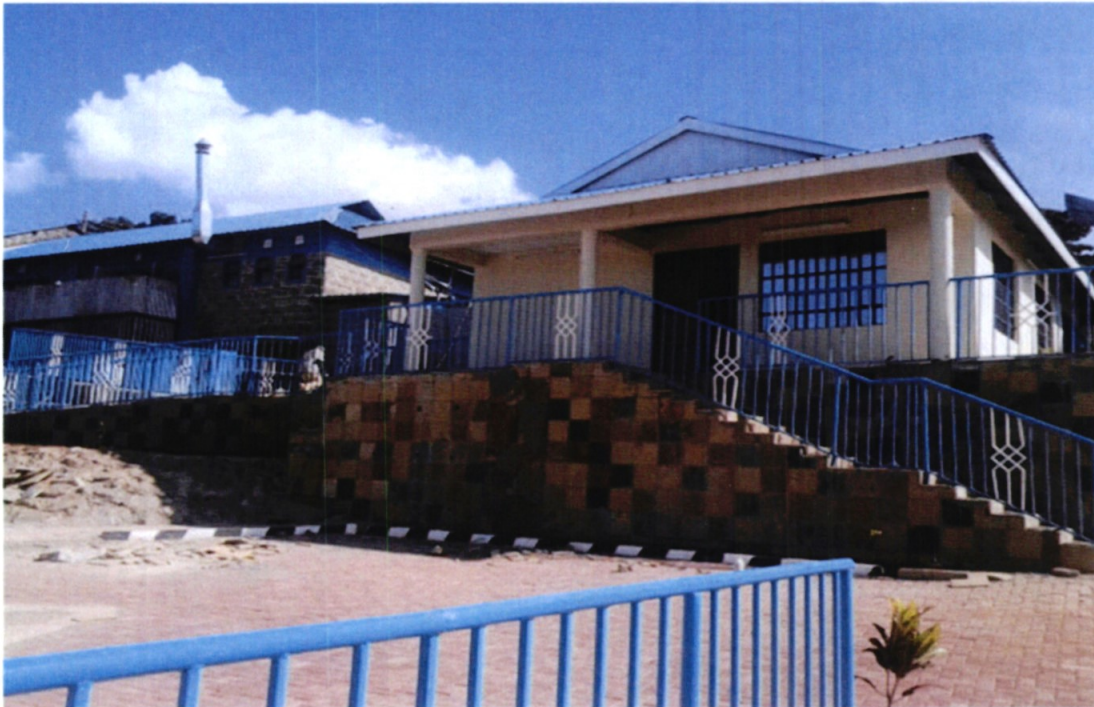
Photo 17: CWSK Muranga Phase 1: – Health Centre (complete)
