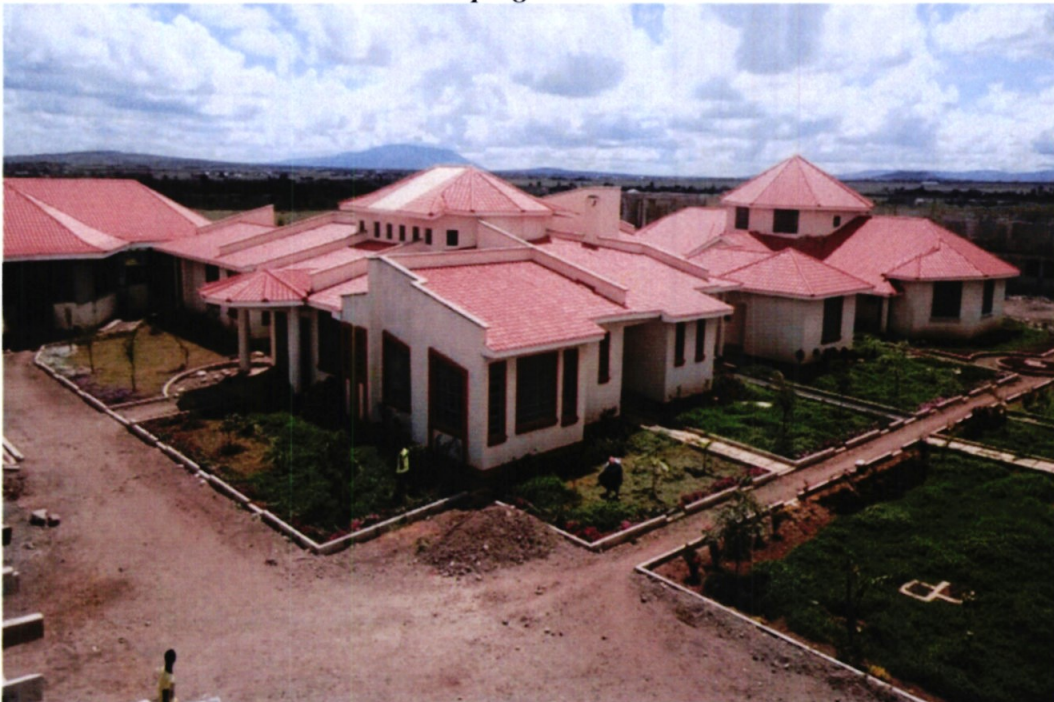
Photo 21: CWSK Joska- Bungalow unit in progress
