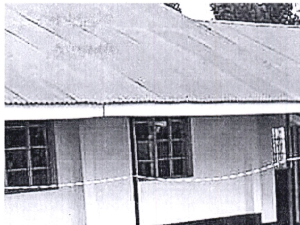
Renovation of 5.No. Classrooms at Kanyimach Primary School.
