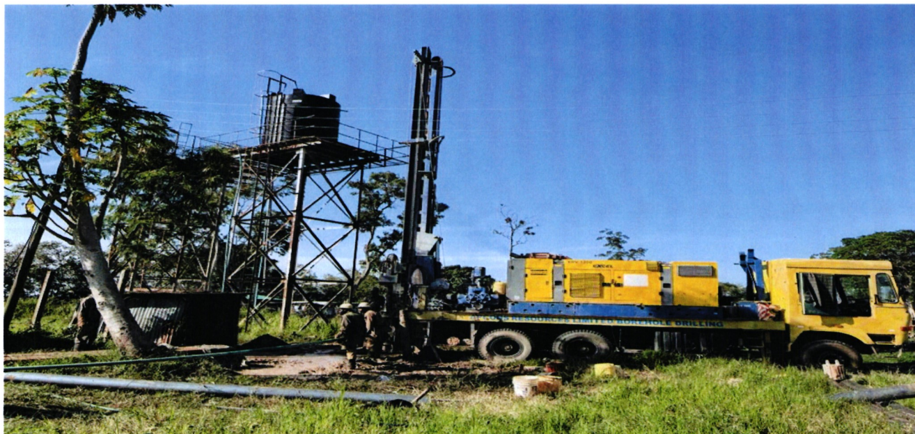
Drilling of a borehole
