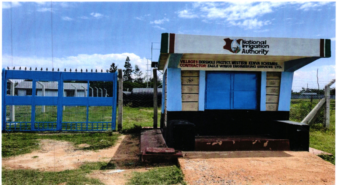
A water access point
