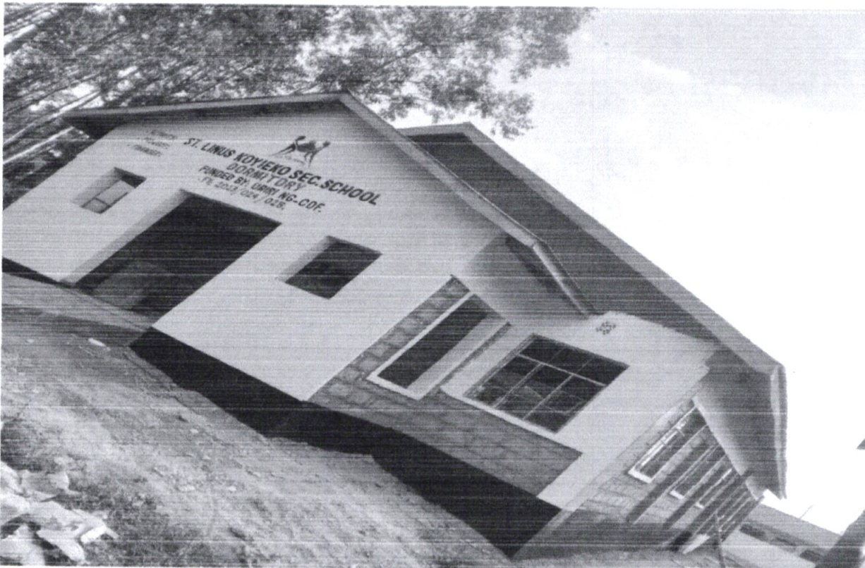
Dormitory at St. Linus Koyieko Mixed Secondary School
