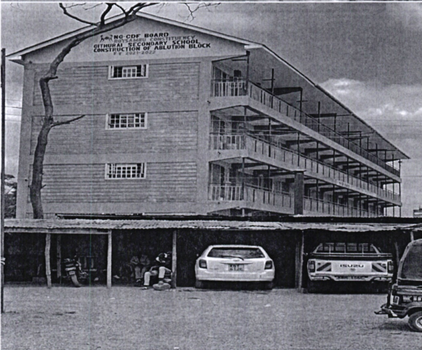
Githurai Secondary School three storey tuition and ablution Block
