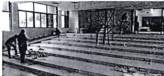
Finishing touches on the new Administration block
