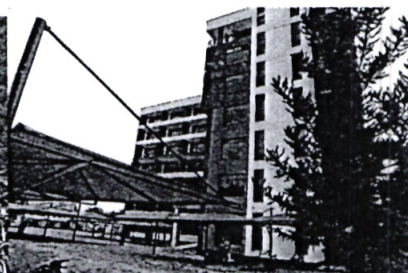
The new Administration block
