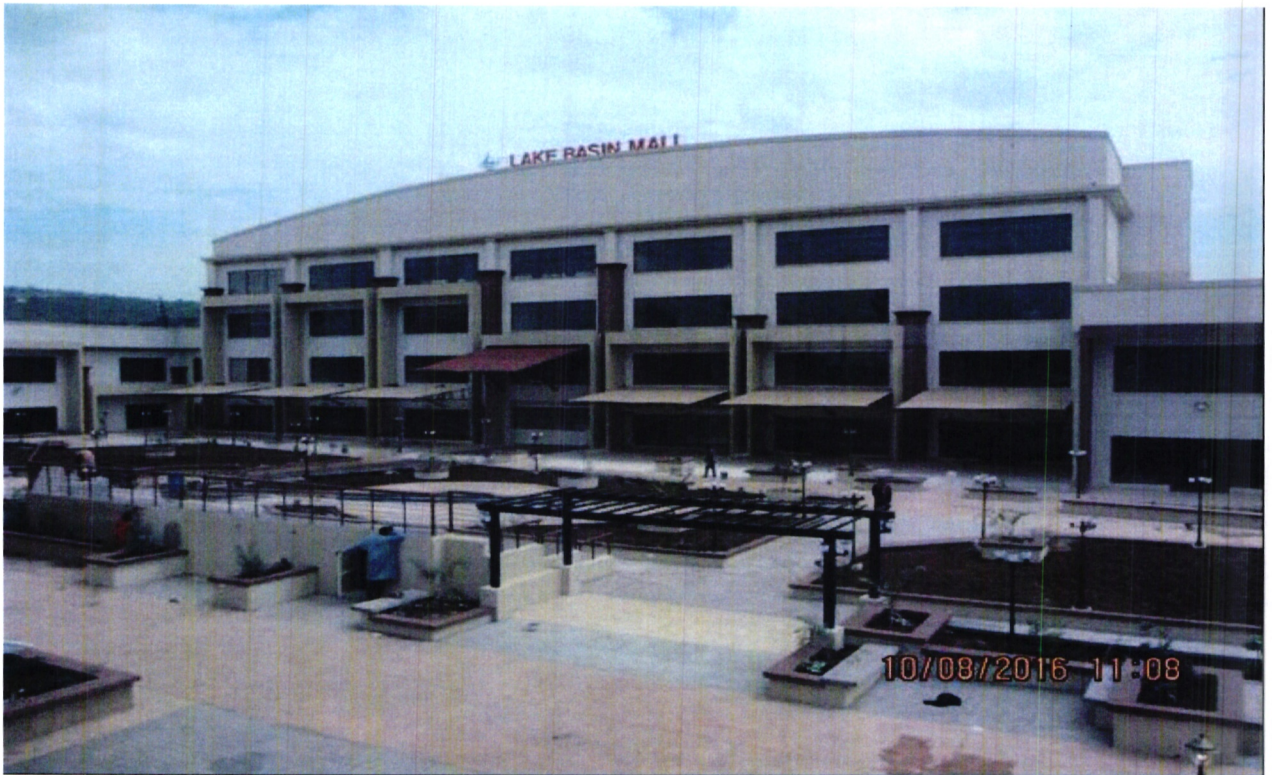
Mall Entrance – Red Canopy
