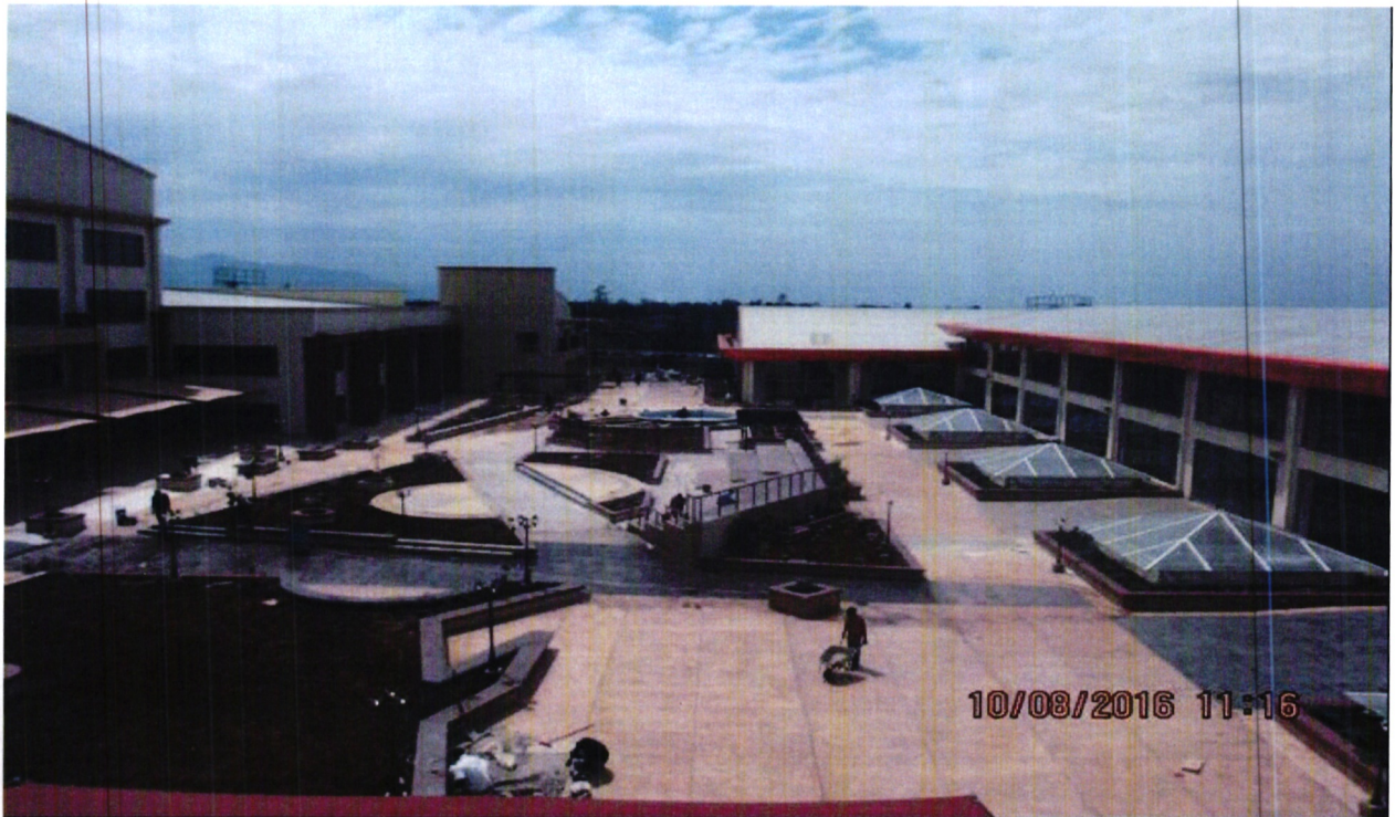
Central Courtyard- Showrooms to the Right
