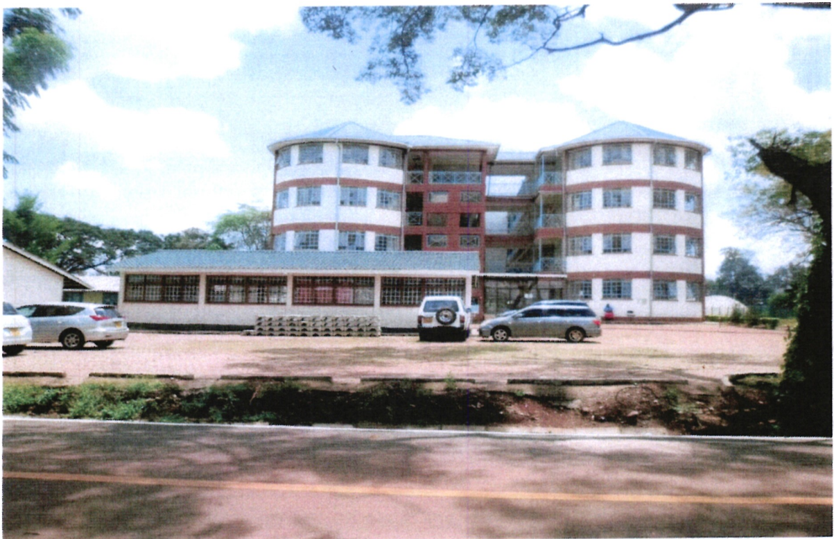
Figure 8: College internal Access roads
