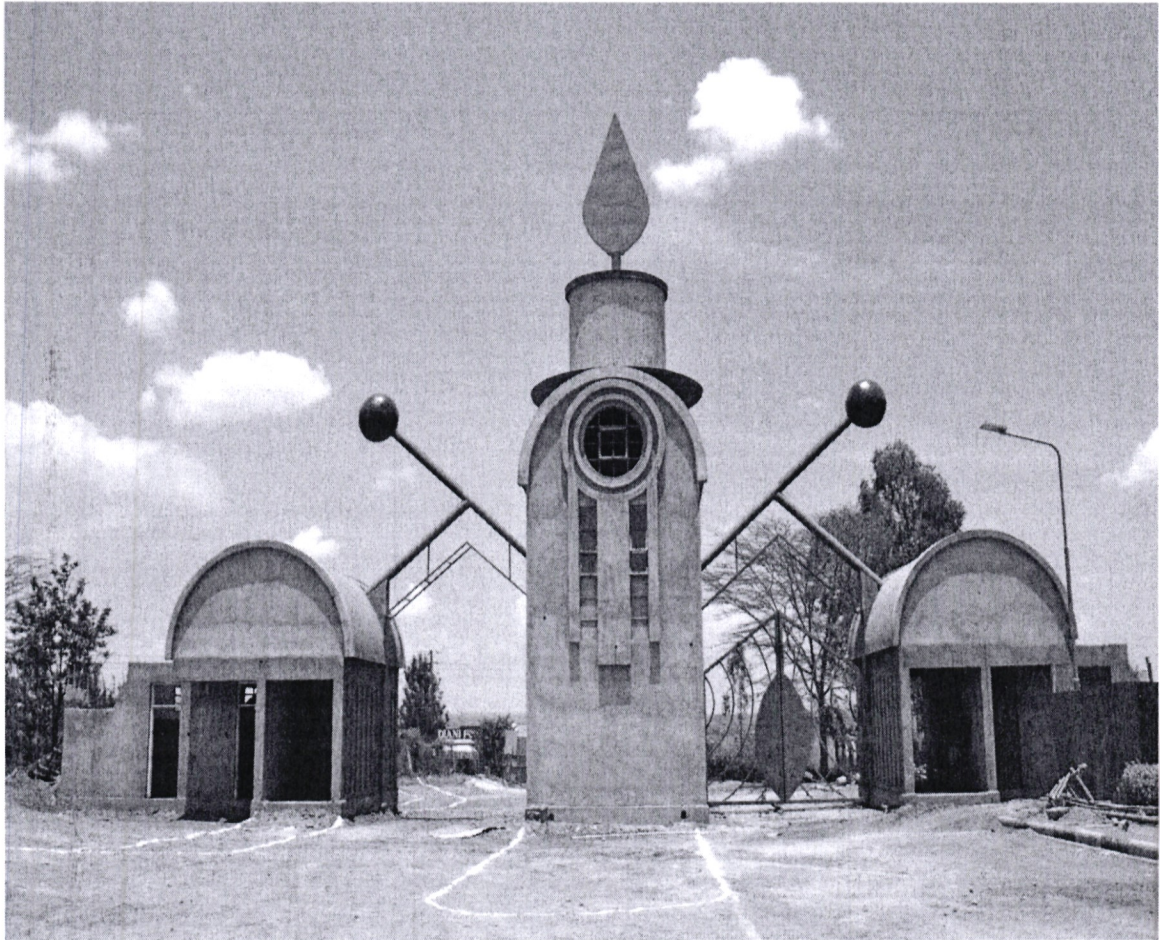
Ongoing construction of the University main gate
