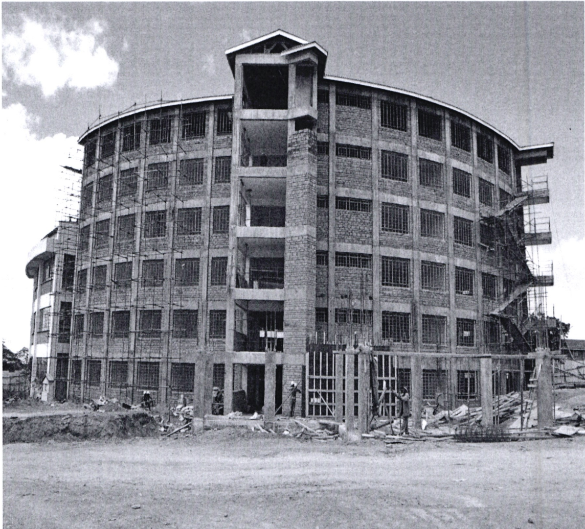
The University Tuition block under construction
