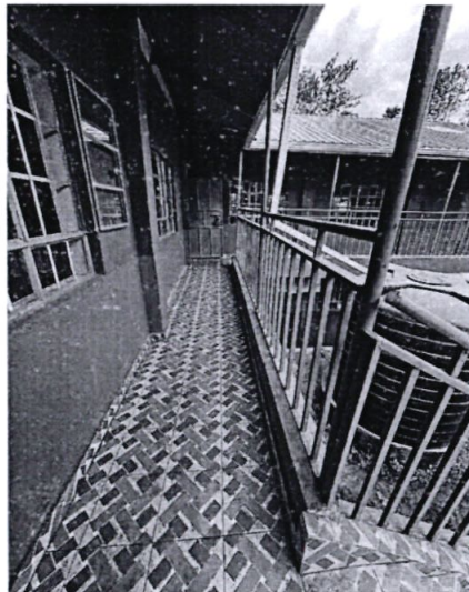
Fig. 1.0–Renovation of 6 No. classrooms at Gakunju Memorial Primary School (FY 2023-2024)
