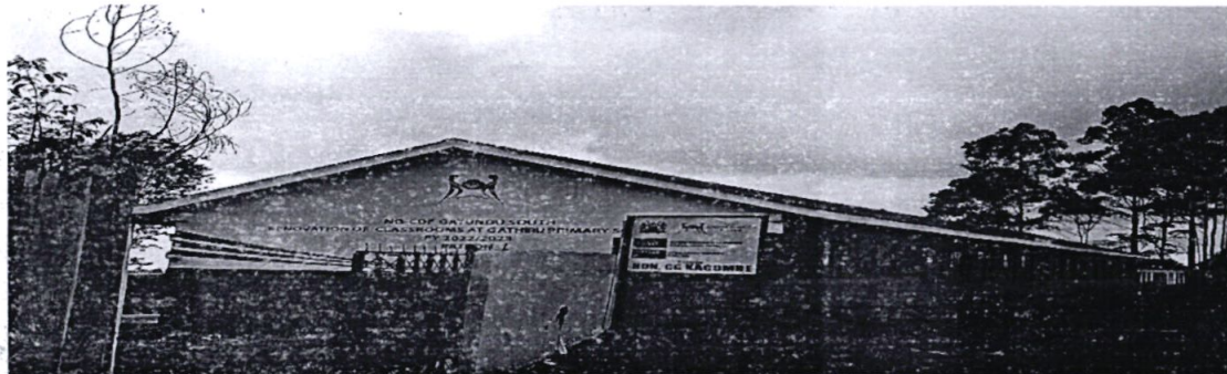
Fig 1.2 Renovation of 6 No. classrooms at Gathiru Primary School (FY 2022-2023)
