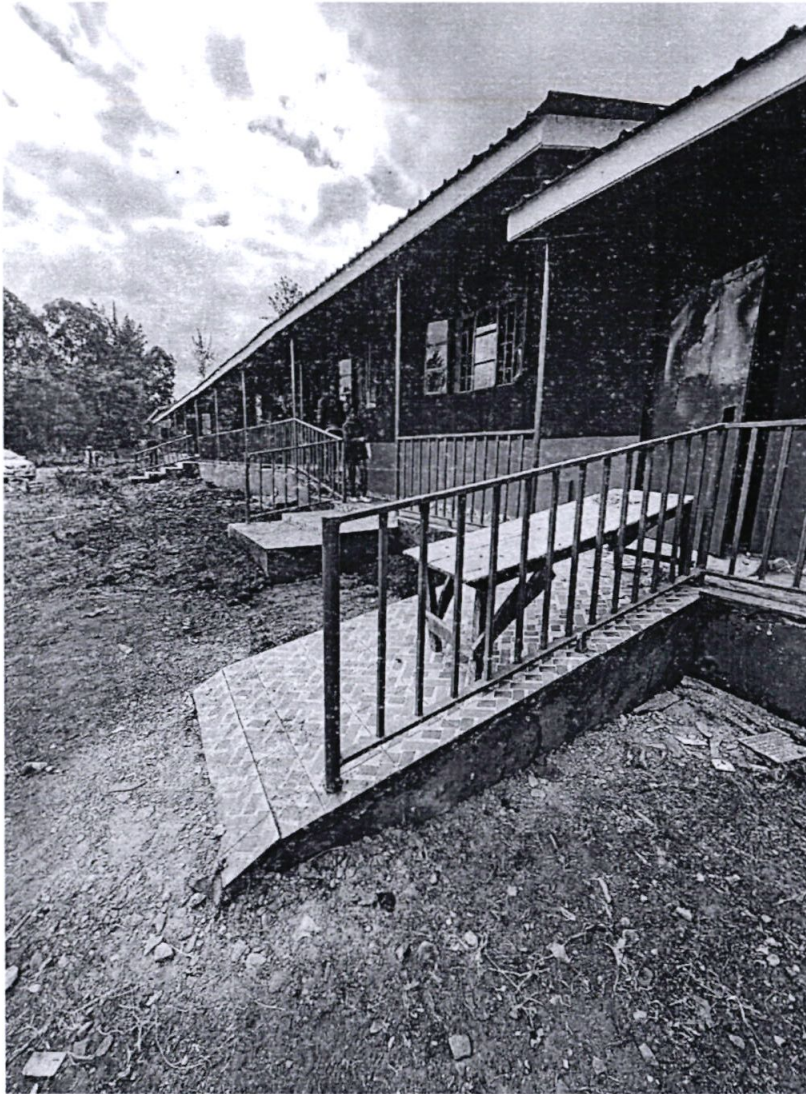
Fig 1.1 Renovation of 6 No. classrooms at Wamitaa Primary School (FY 2023-2024)
