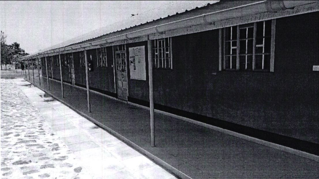
Pic 3: Four new classrooms at Kombewa KMTC
