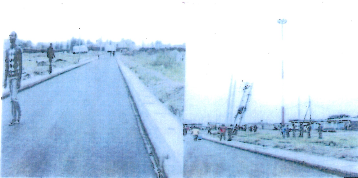
Roads, footpaths and high mast lighting installed in Informal settlements
