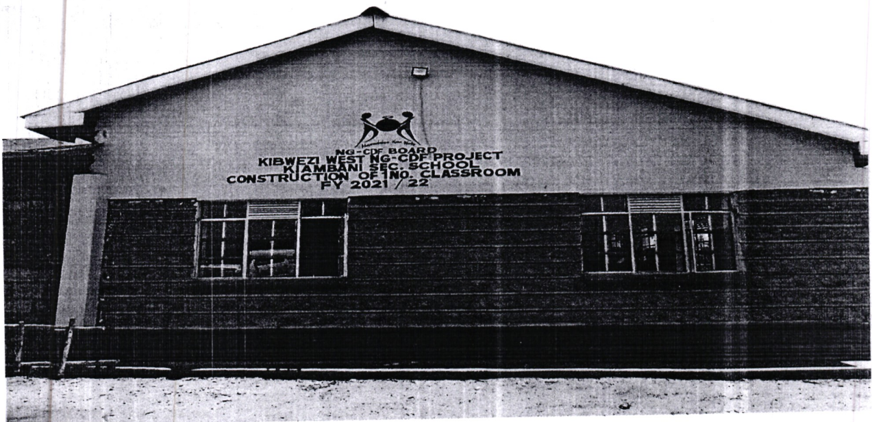
KIAMBANI SECONDARY SCHOOL-ONE CLASSROOM FY 2021/2022
