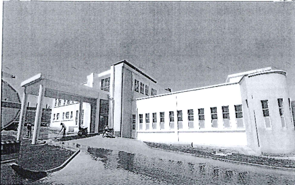
Figure 4: Newly Constructed MARWASCO Office Block
