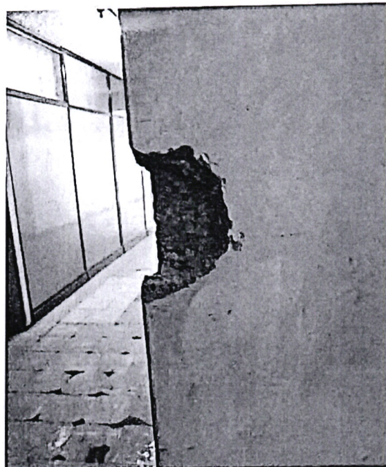
Photo showing plaster cuttings on columns and beams reported to have been done by EACC officers for during their investigations.
