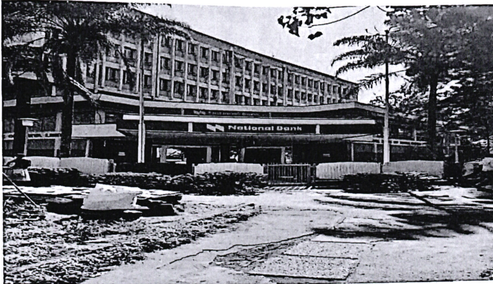
Photo showing frontage of the National Bank building, and the area of road reserve to boundary fence.
