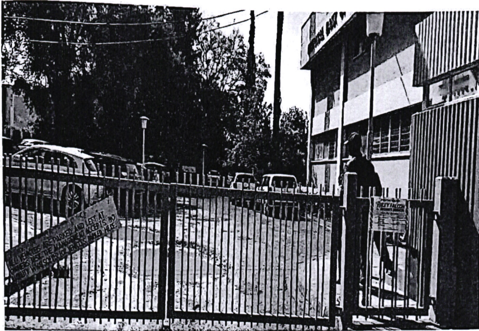
Photo showing entrance gate to the parking area from Ronald Ngara Road and the potholes on the access road and parking.
