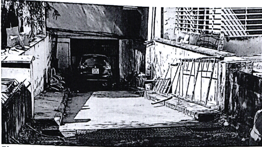
Photo showing access to the basement parking.
