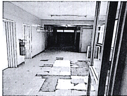
Photo showing worn out floor tiles on 1 st and 2 nd floors.
