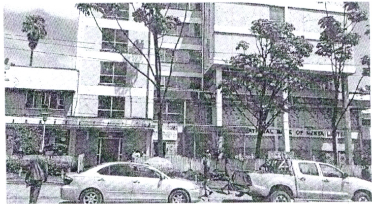
Building view from across Oloo Street
