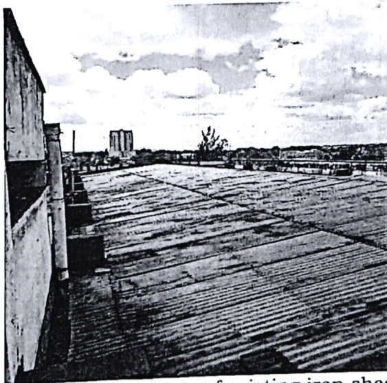
Photo showing state of existing iron sheets roofing.
