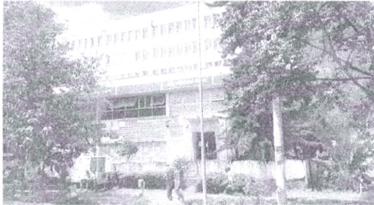
Building view from across Uganda road
