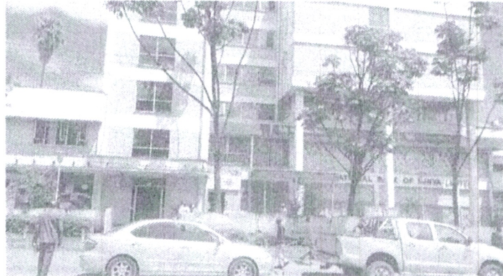
Building view from across Oloo street
