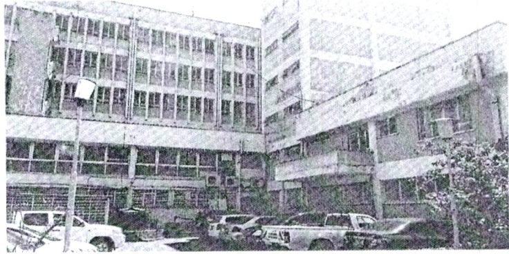
Rear view from KVDA Building
