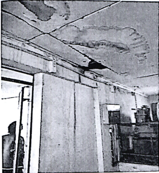
Photo showing damage caused on ceiling and walls by leaking water.
