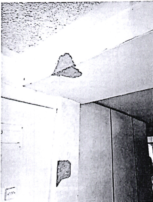
Photo showing plaster cuttings on columns and beams reported to have been done by EACC officers for during their investigations.
