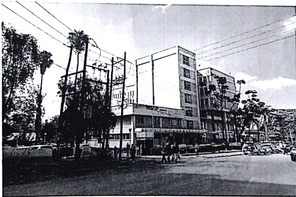
Photo showing the view of the building from Ronald Ngara Road.
