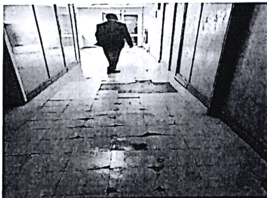
Photo showing worn out floor tiles on 1 st and 2 nd floors.
