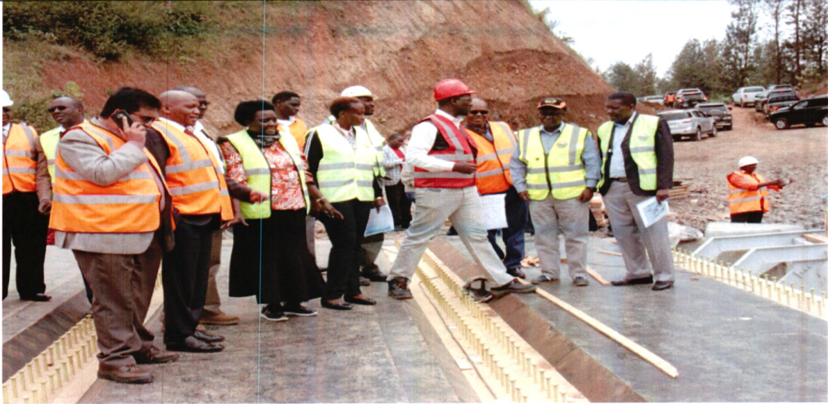
Figure 5: Board Members and management conducting an inspection of the Meru Bypasses projects.
