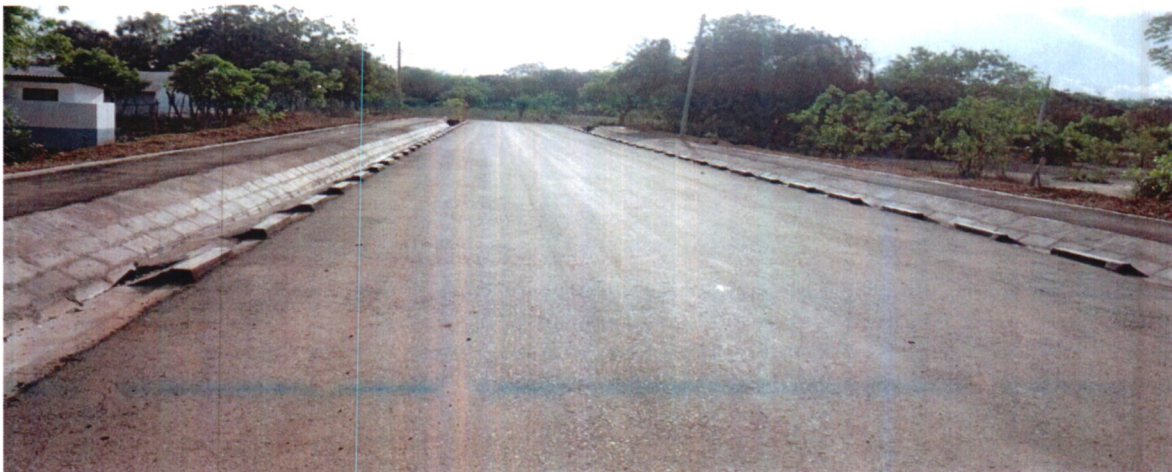
Figure 6: Ongoing construction of Mokowe Township Roads in Lamu County
