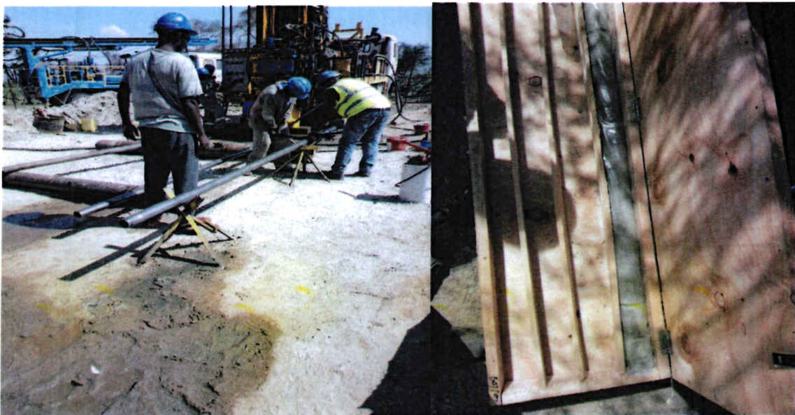
Drilling of stratigraphic wells in Block 14T, Tertiary Rift Basin
