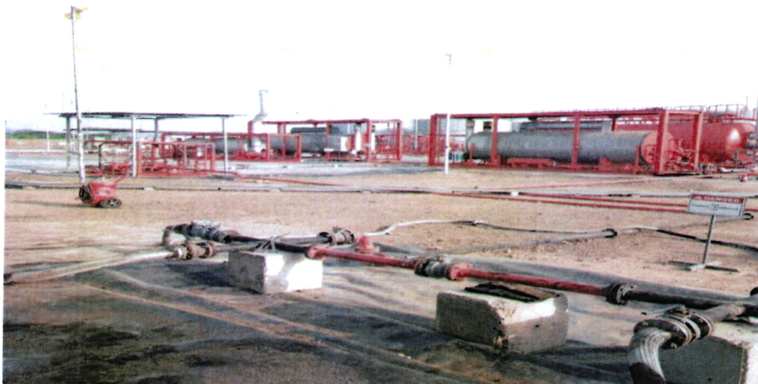
EOPS Facilities (Separator) being Decommissioned
