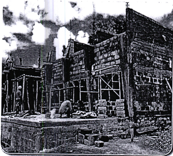
Ongoing Nyahururu Railway Station
