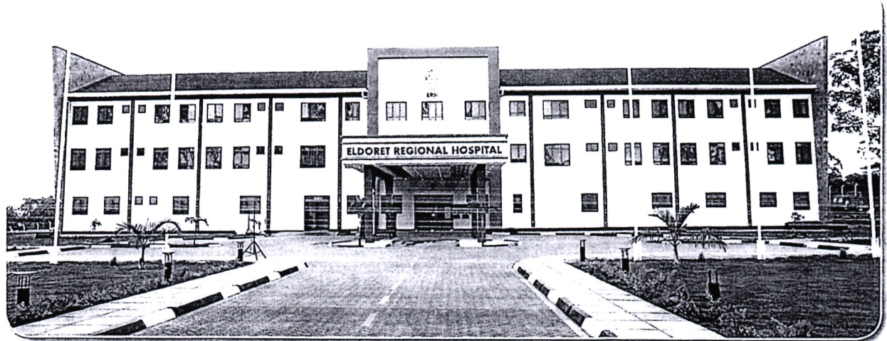
Front view of the completed Eldoret Regional Hospital (ERH) at Moi Barracks as at 30 June 2022
