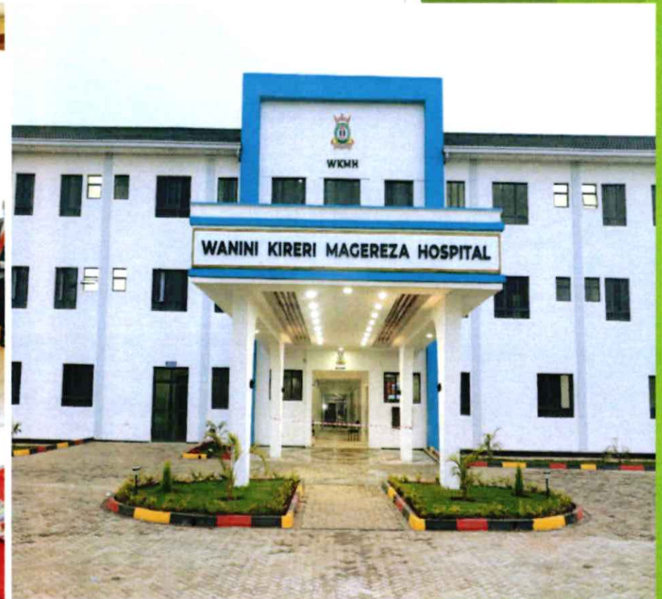
Construction and equipping of the Magereza Hospital is 100% complete. 271 Health care workers have been recruited and deployed. The aim is to enhance the provision of healthcare to staff, inmates, and their families.
