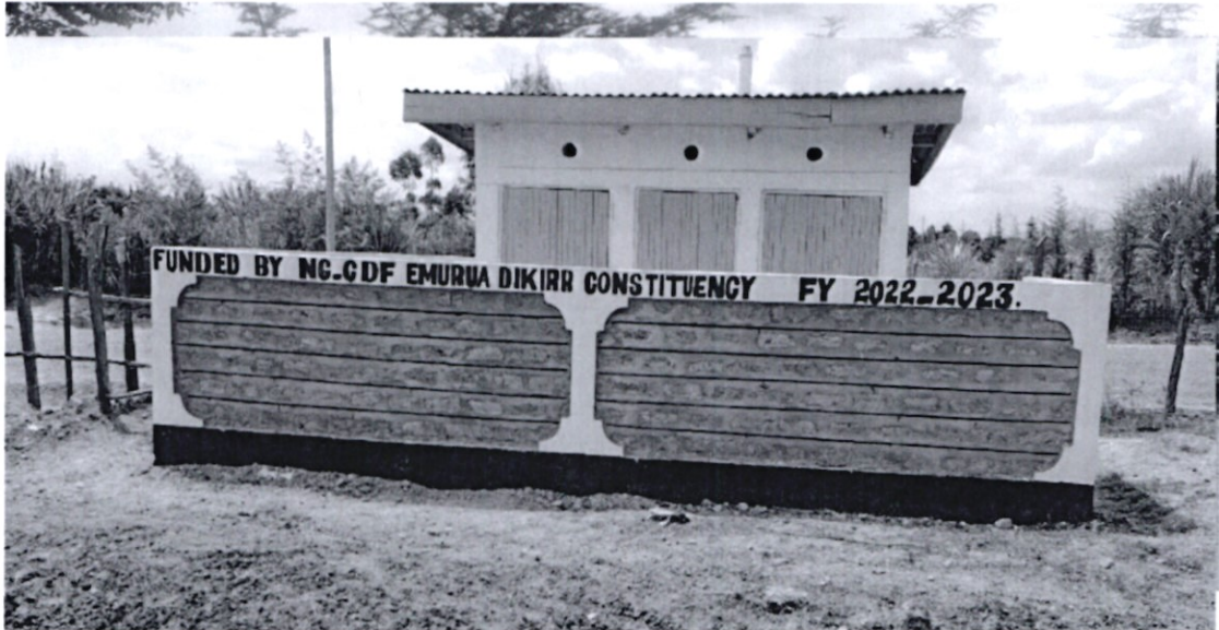
Emergency pit latrines funded in financial year 2022/2023
