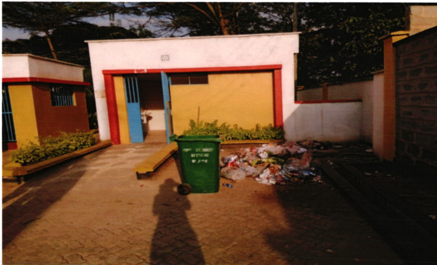
Annexure 10A: Improper Waste Management Kisumu Social Hall
