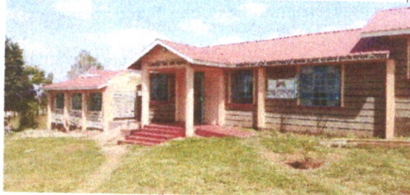
Korrinko secondary school- administration
