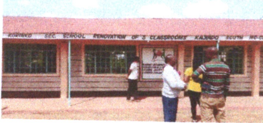
Korinko Secondary School- Renovations
