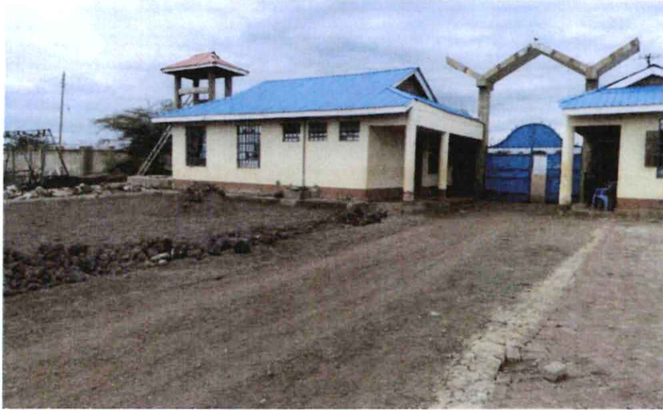
Photo 19: CWSK Isiolo TPS: Health Centre, Guard house and reception office
