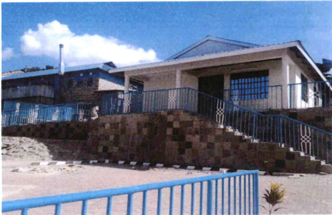
Photo 21: CWSK Muranga Phase 1: – Health Centre (complete)
