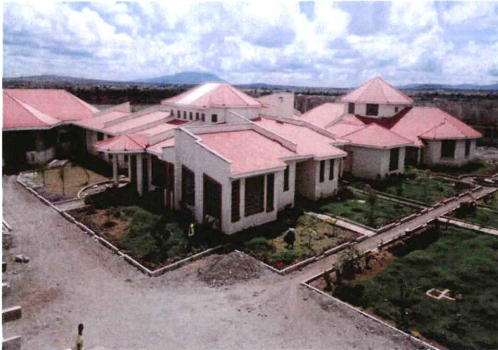
Photo 25: CWSK Joska: Bungalow unit in progress
