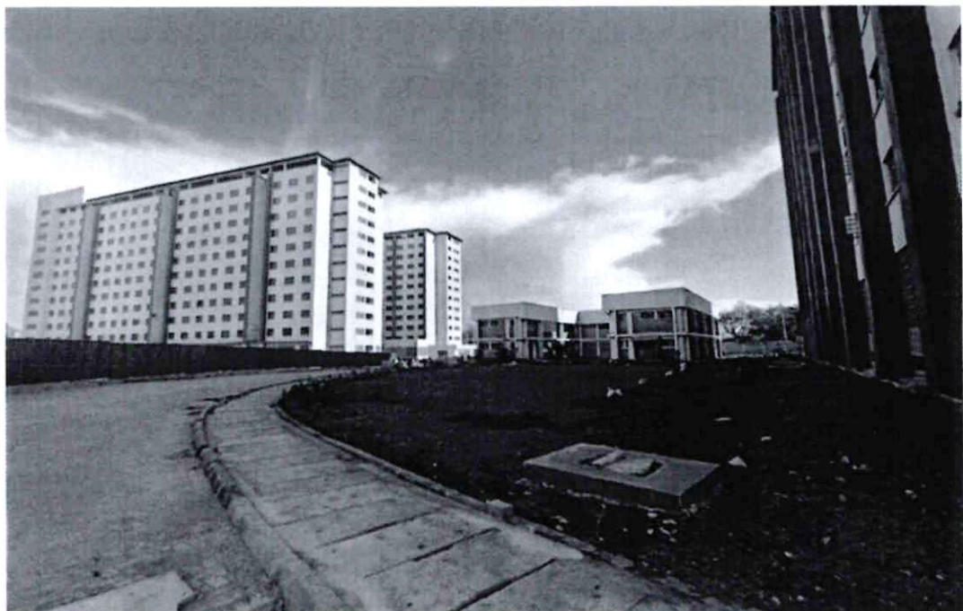
Progress of Phase I of Housing Makasembo Project.
