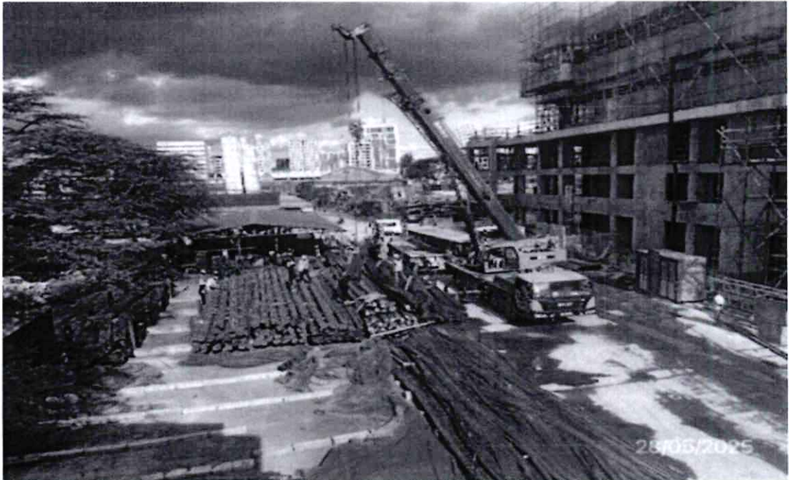
Source: Clerk of Works Report - Reinforcement offloading on site
