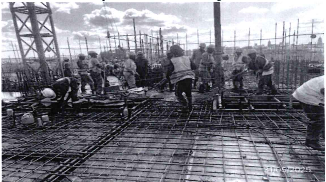
Source: Clerk of Works - Block A1-5th floor slab concrete works
