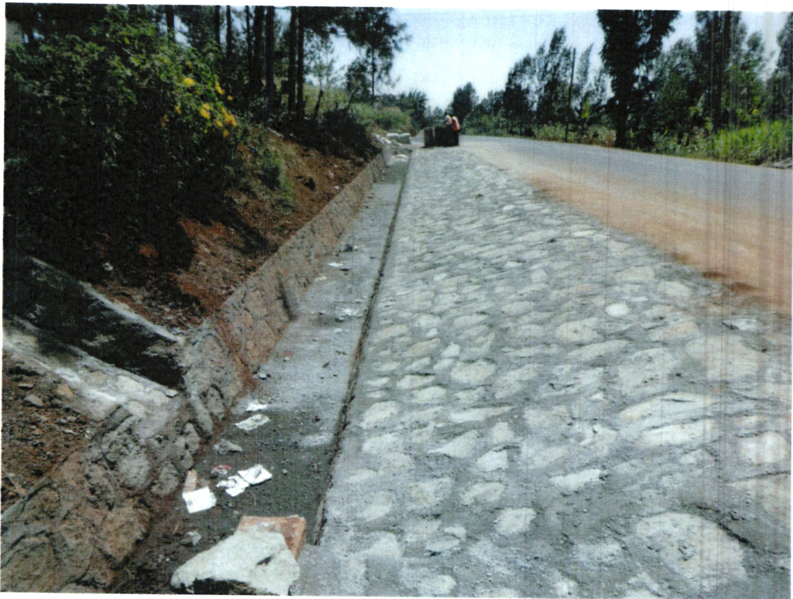
Protection Works on Gatundu- Karinga -Flyover Road in Kiambu County
