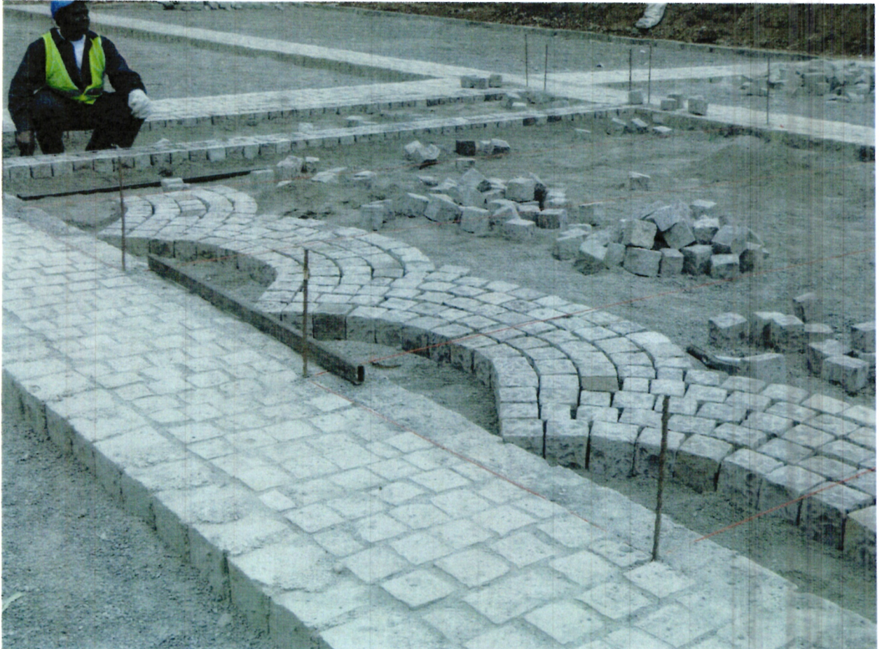
Use of cobblestones as an alternative road surfacing
