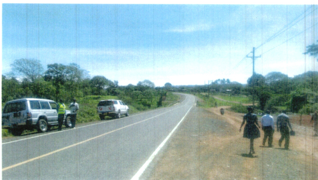
Completed section of rehabilitated Kabenes-Kachibora Road Uasin Gishu
