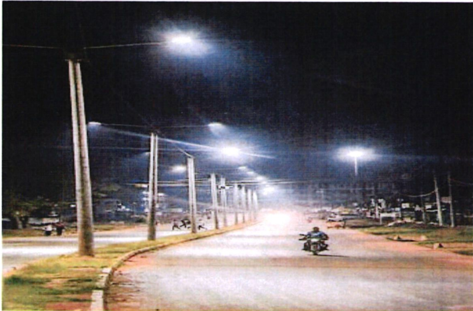
Figure 4: 6.5km Sangalo Junction – Kanduyi Dual carriageway
