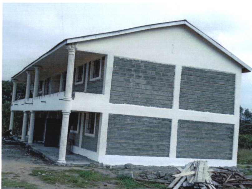
Highway Secondary School (Construction of 4 classrooms)
