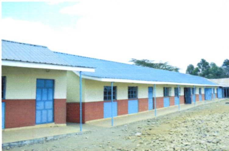
Karima Primary School (Renovation and upgrading of 8 classrooms)
