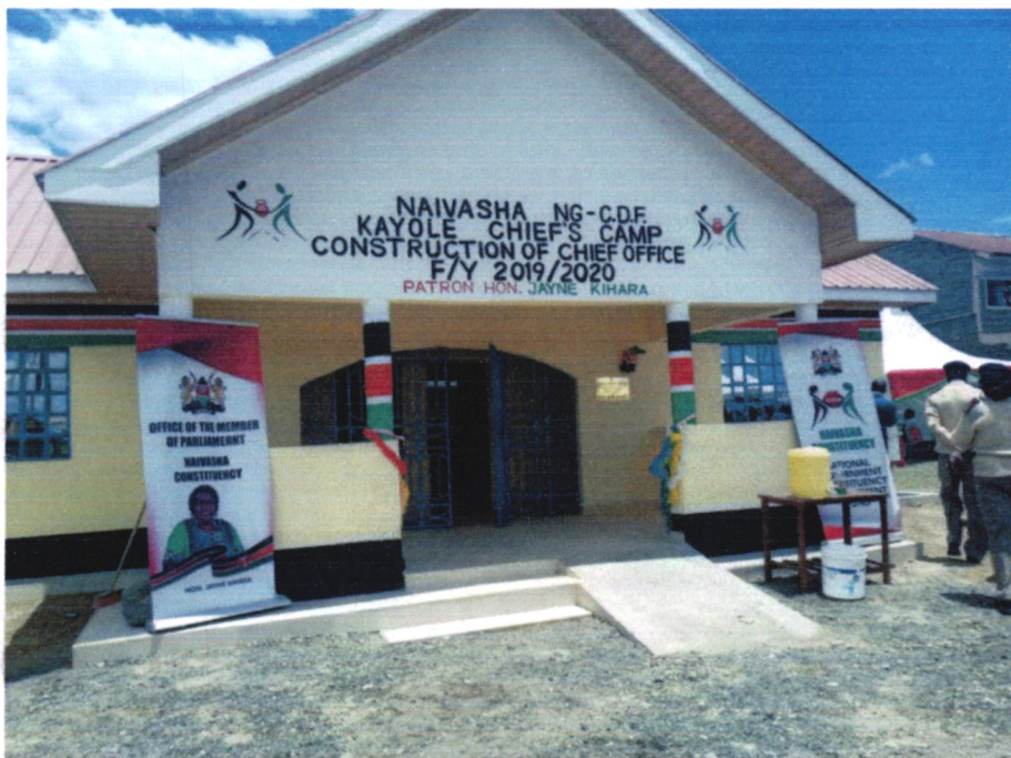
Kayole Chiefs office (Construction of a 3 roomed office)
