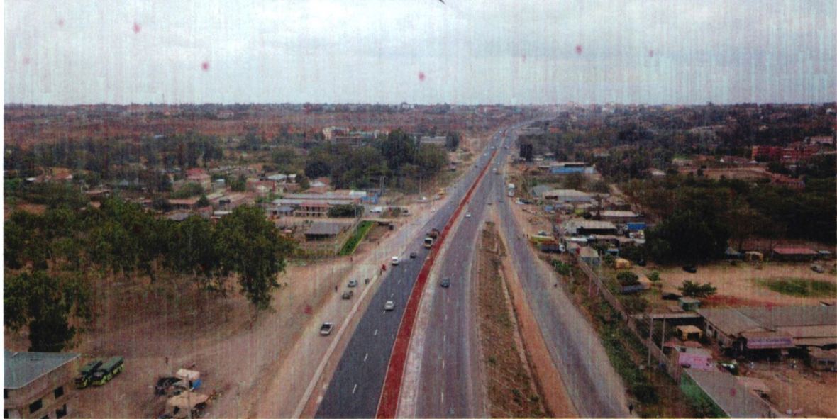
Figure 1: Completed section of Eastern Bypass
