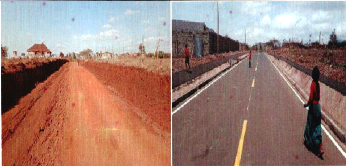
Figure 9: Marsabit town roads-before and after
