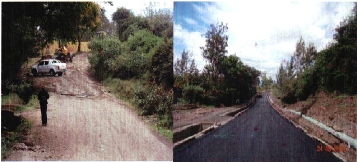
Figure 3: Maragoli Road in Nakuru county before and during upgrade under Low Volume seal programme
