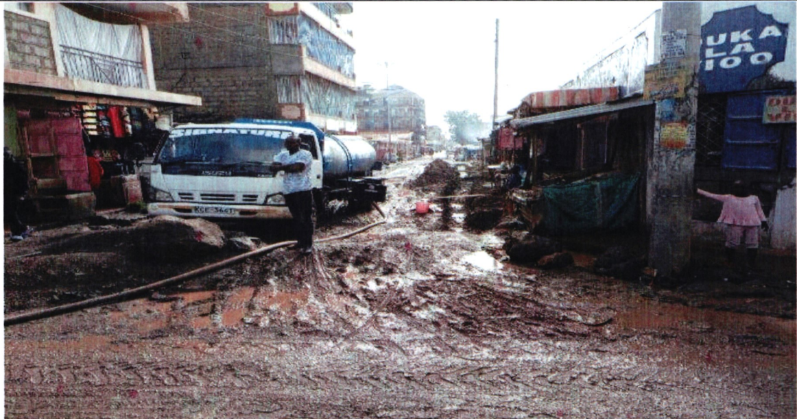
Figure 4: Saika/Omega Road in Dandora Nairobi county before upgrade
