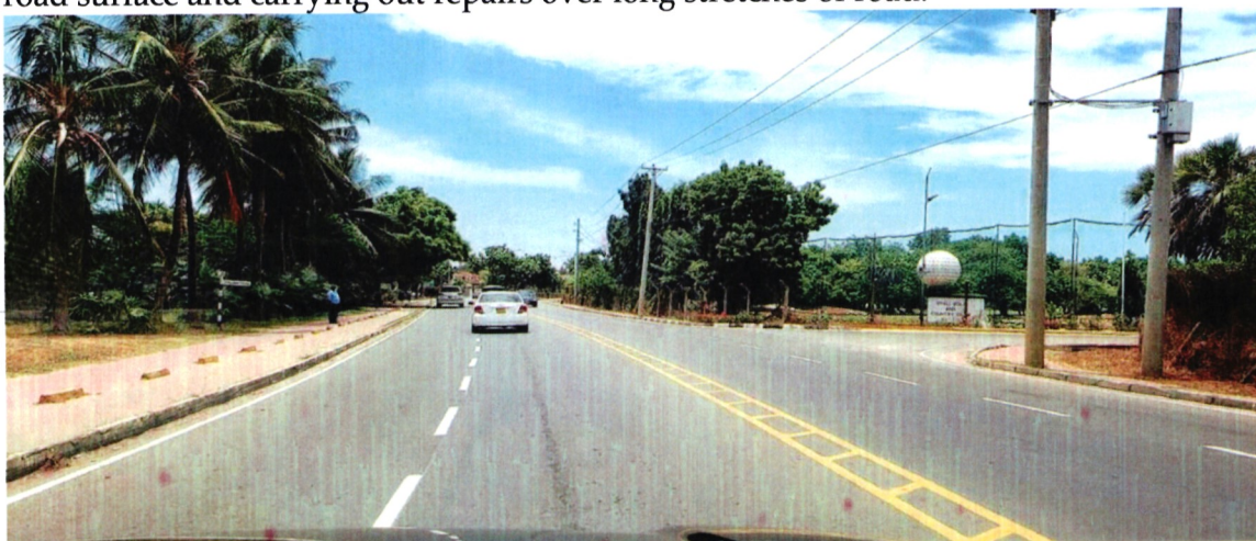
Figure 10: Rehabilitation of Links Road Nyali , Mombasa County
