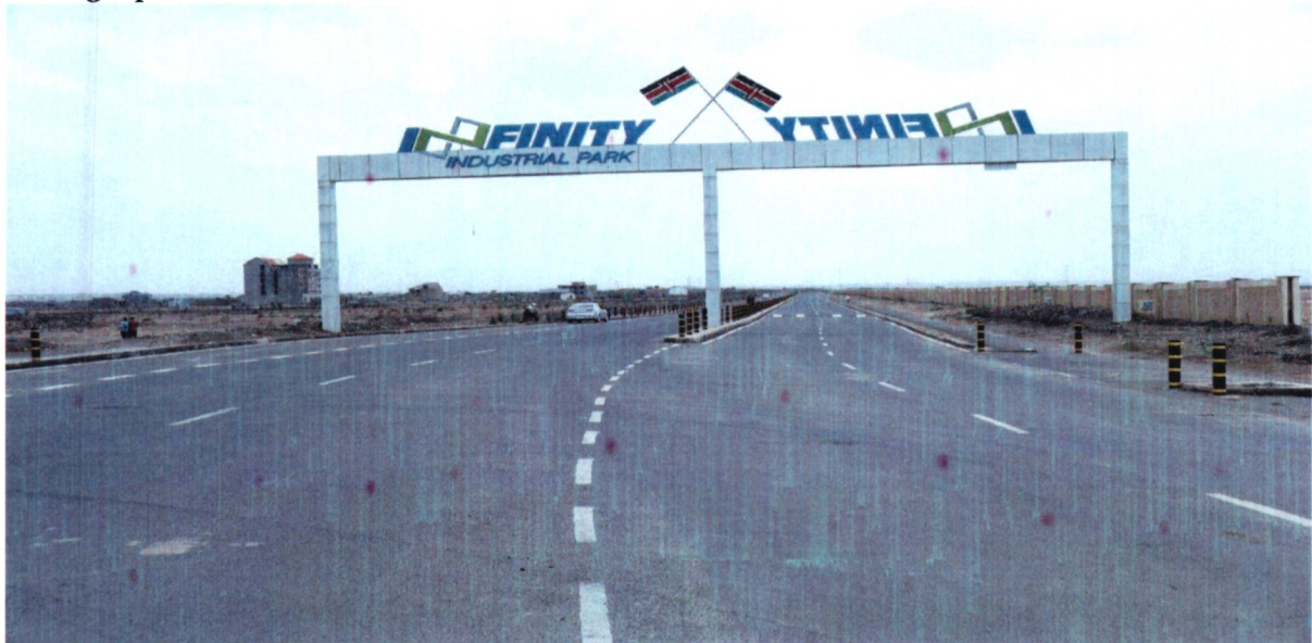
Figure 6: Completed section of Infinity park roads
