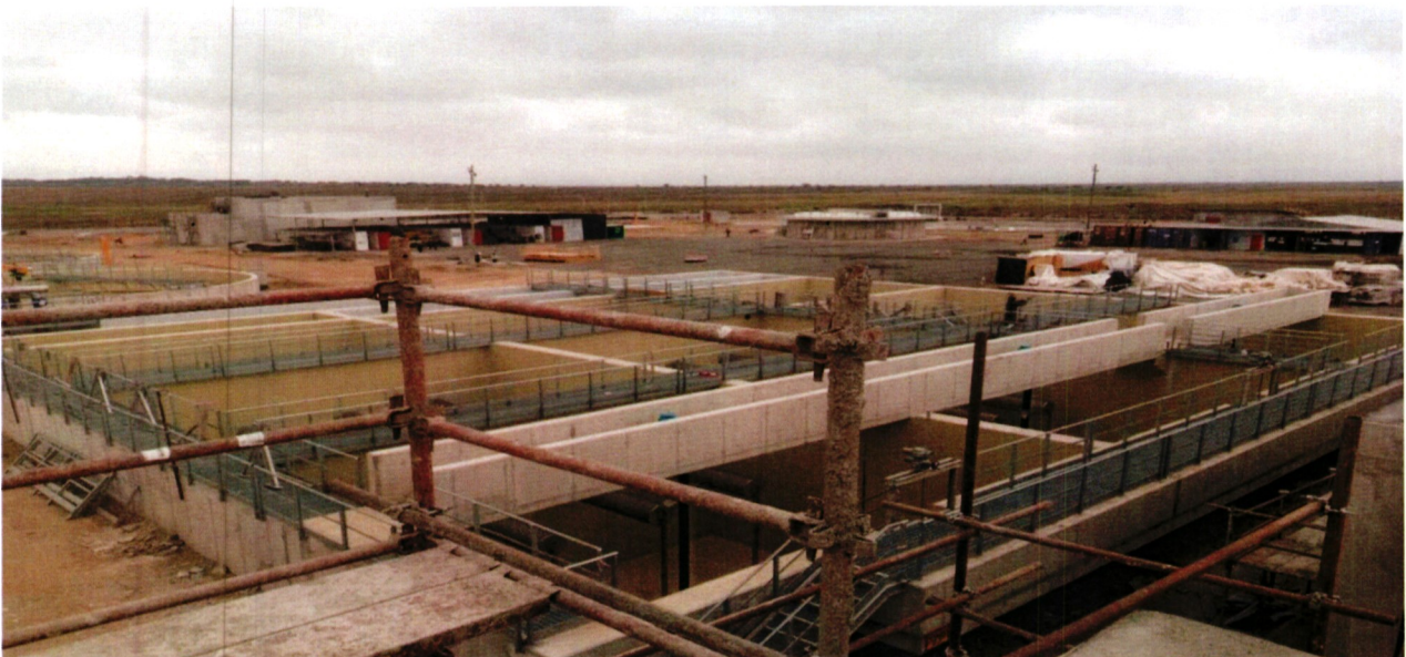
MBBR tank under construction
