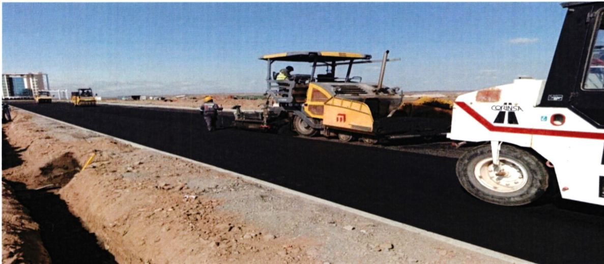
Asphalt laying at LR01
