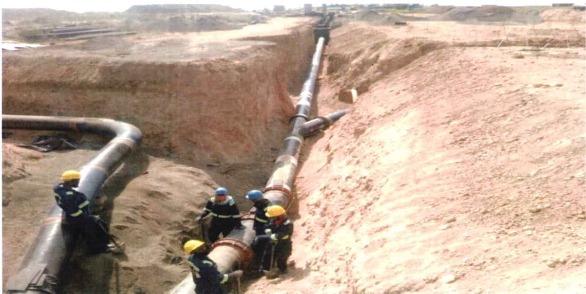
Pipe laying for Solid Waste network along Green Transit Corridor
