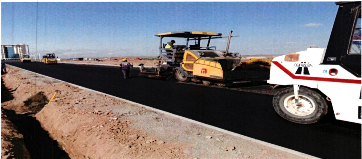
Asphalt laying at LR01
