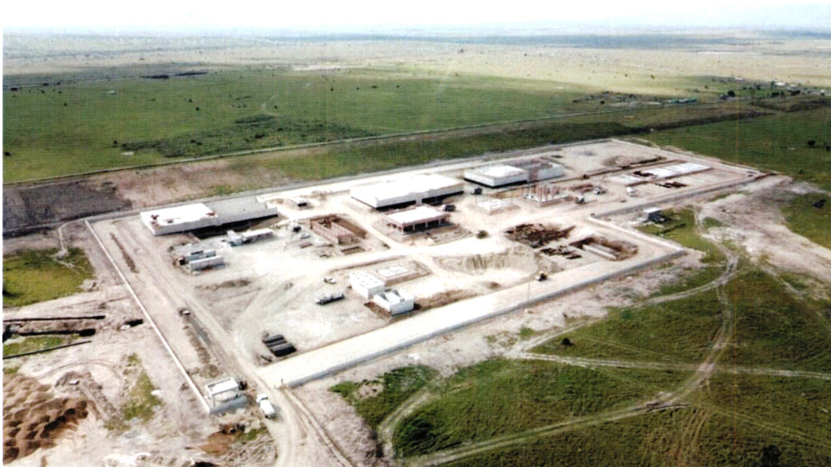
Water Treatment under Construction
