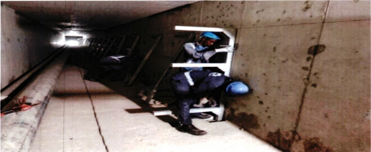
Installation of Utilities Racks inside Tunnel C situated along Auto boulevard.
