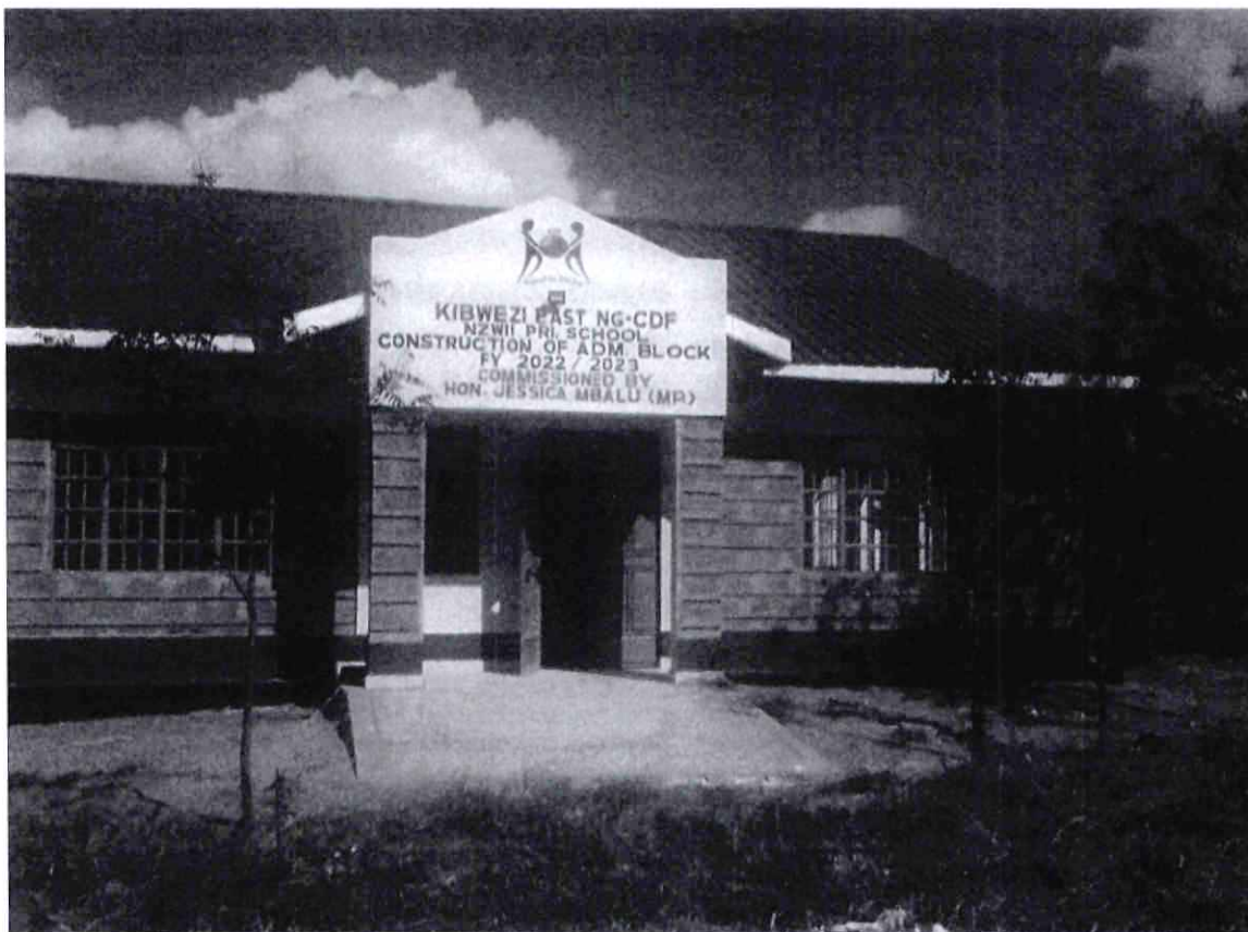
Project name: Nzwii Primary School Activity : Construction of administration block
