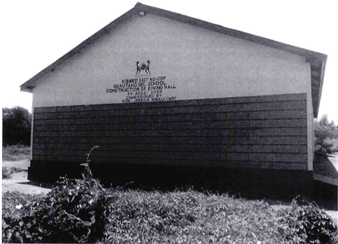
Project Name: Makutano Secondary School Activity : Construction of dining hall
