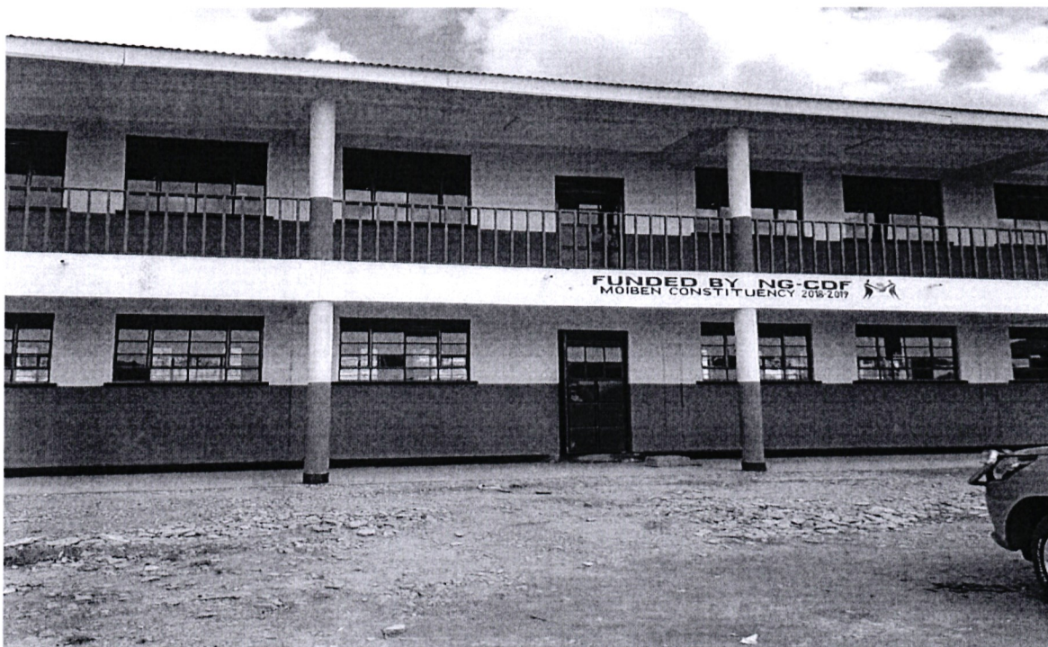
Ngomongo primary school- Constructed classrooms.
