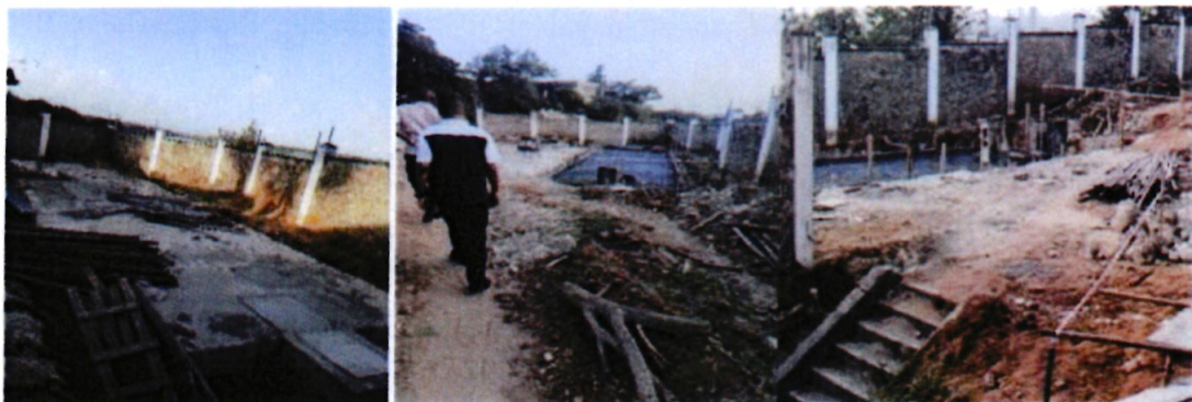
The Survival Training and Certification Centre Project site
