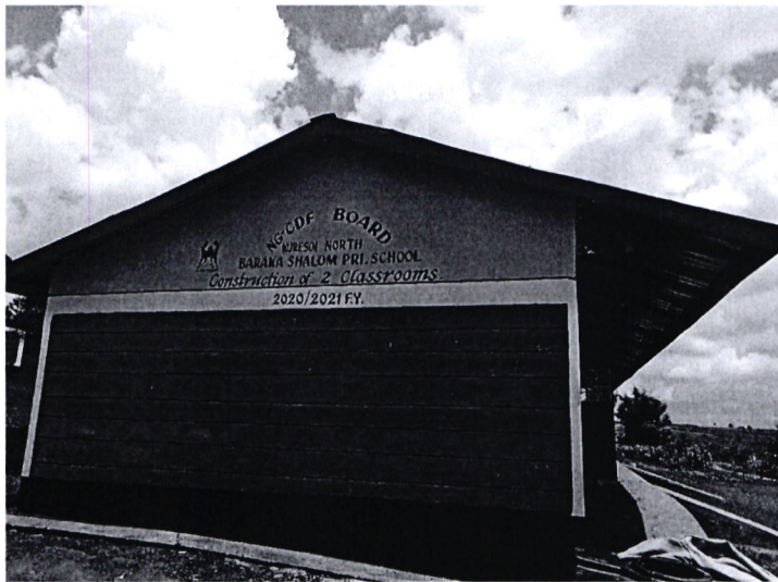
Baraka Shalom Primary School-2 Classrooms-Kamara Ward
