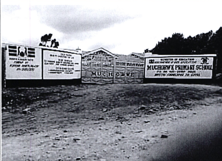
Muchorwe Pri School-Construction of main gate/fencing-Kamara Ward
