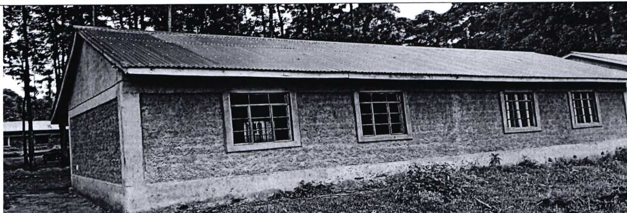
KEIGAMERE PRIMARY SCHOOL – CONSTRUCTION OF 2 CLASSROOMS
