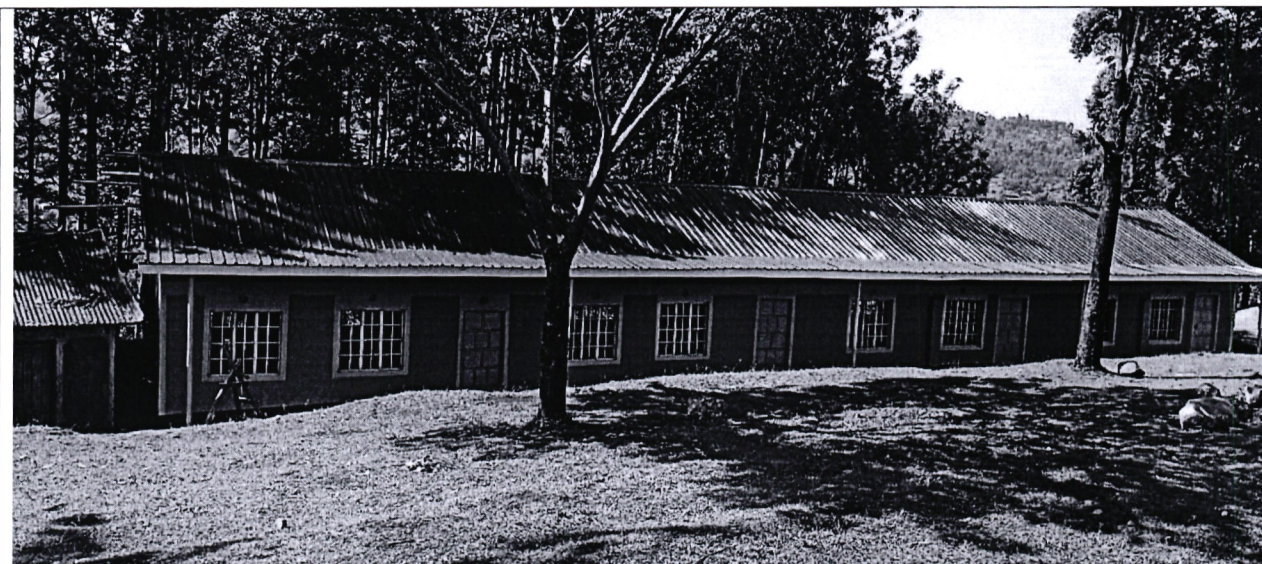
RENOVATED 4 CLASSROOMS AT NYAMOKENYE PRIMARY SCHOOL
