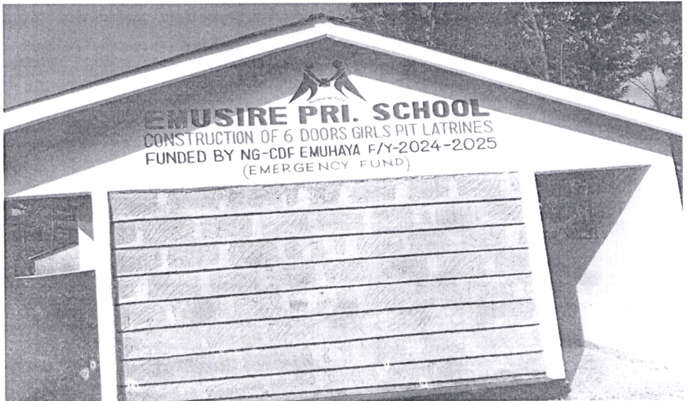
EMUSIRE PRIMARY SCHOOL –Construction of 6 door Pit Latrine at Kshs 600,000
