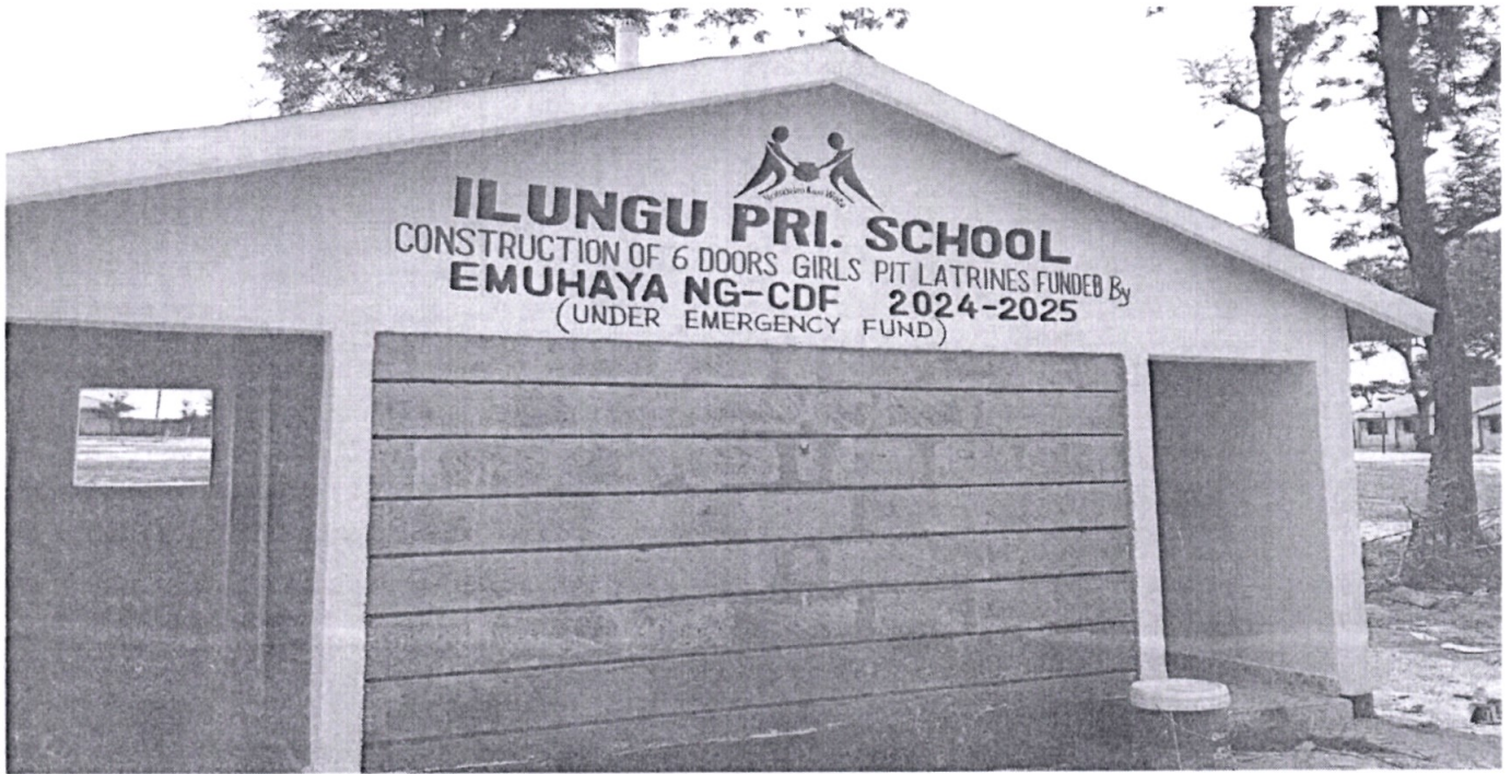
ILUNGU PRIMARY SCHOOL - Construction of 6 door Pit Latrine at Kshs 600,000
