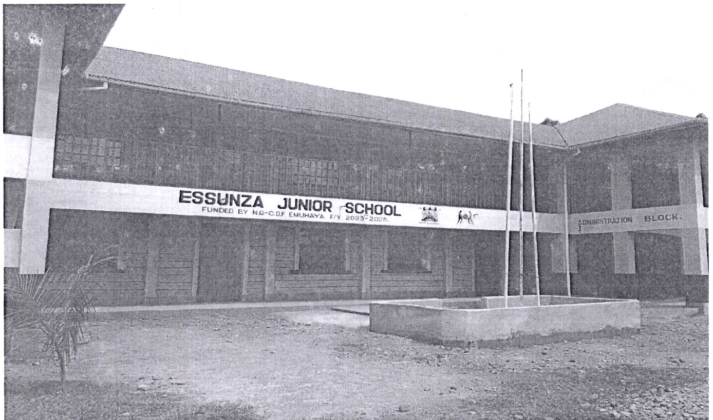
ESSUNZA PRIMARY SCHOOL- construction of a storey block consisting of 7 classrooms
