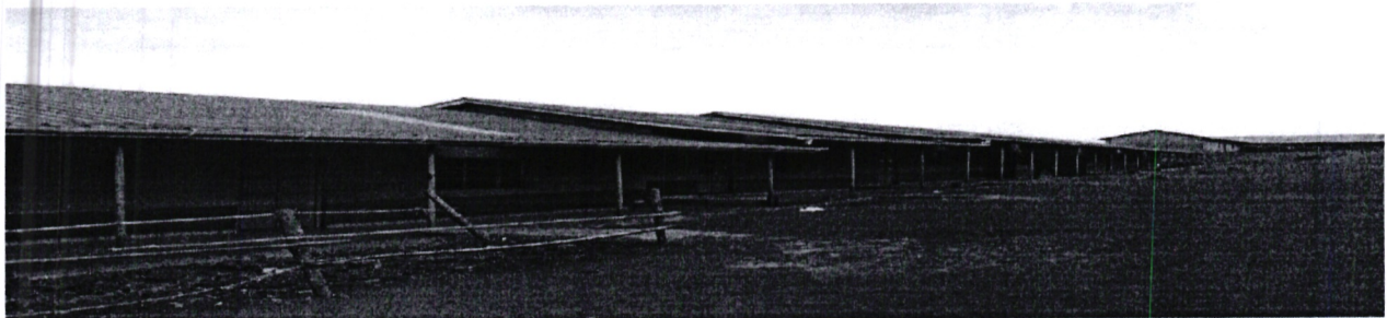
CHANIA WARD, KANJUKU PRIMARY SCHOOL: RENOVATION OF 9NO CLASSROOMS TO COMPLETION. F/Y 2021/2022
