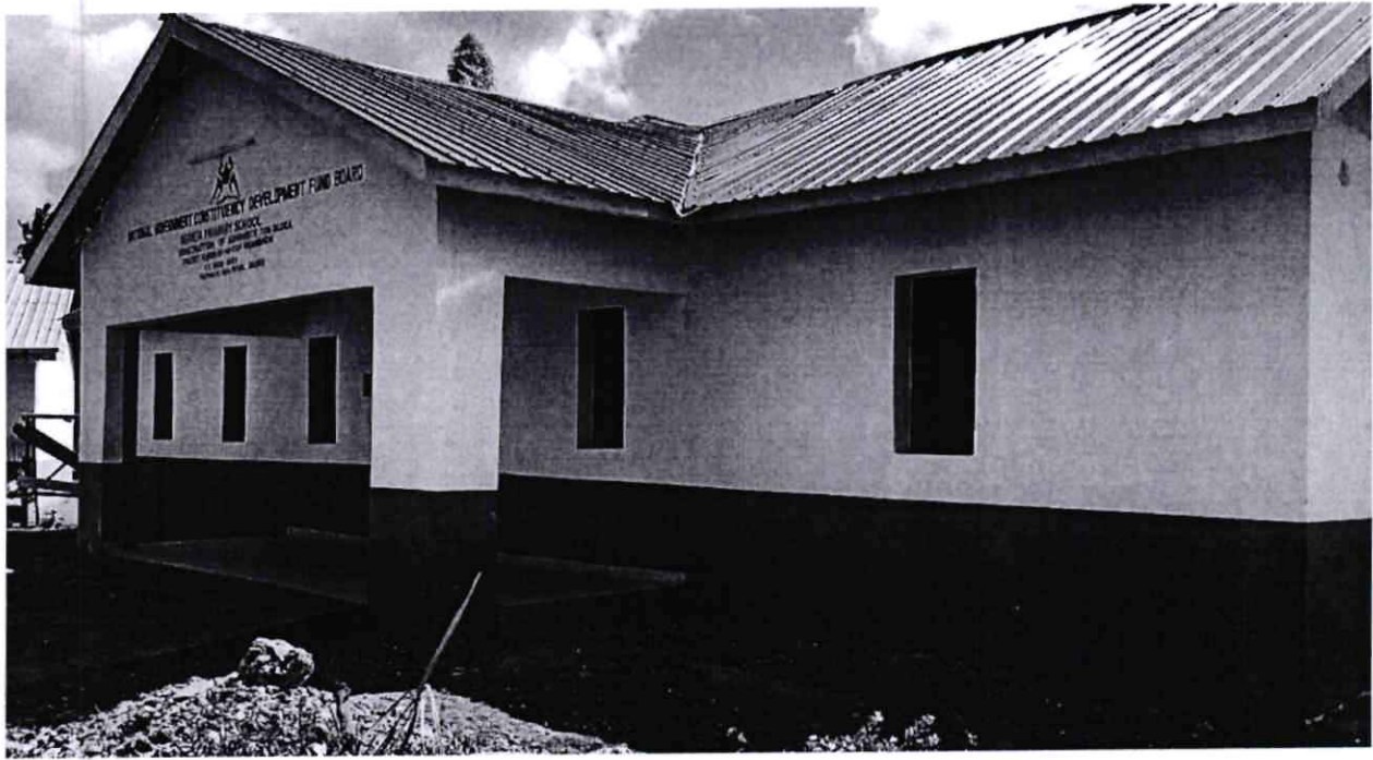
Nganja Primary School; Construction of Administration Block.
