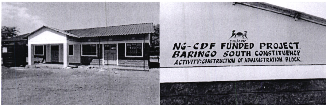
FIG 1.2: Iingarua Pry School new administration block constructed by NGCDF baringo south . FY 2016/2017
