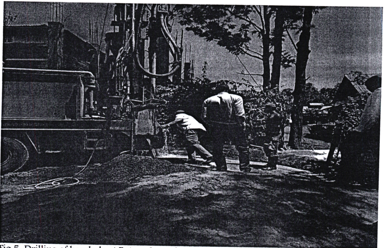
Fig 5. Drilling of borehole at Botoro Secondary School
