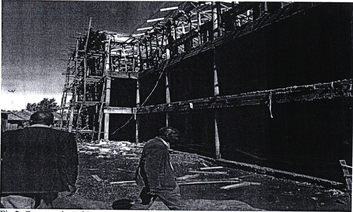
Fig 2. Construction of 2 storey tuition block at Suneka Primary School
