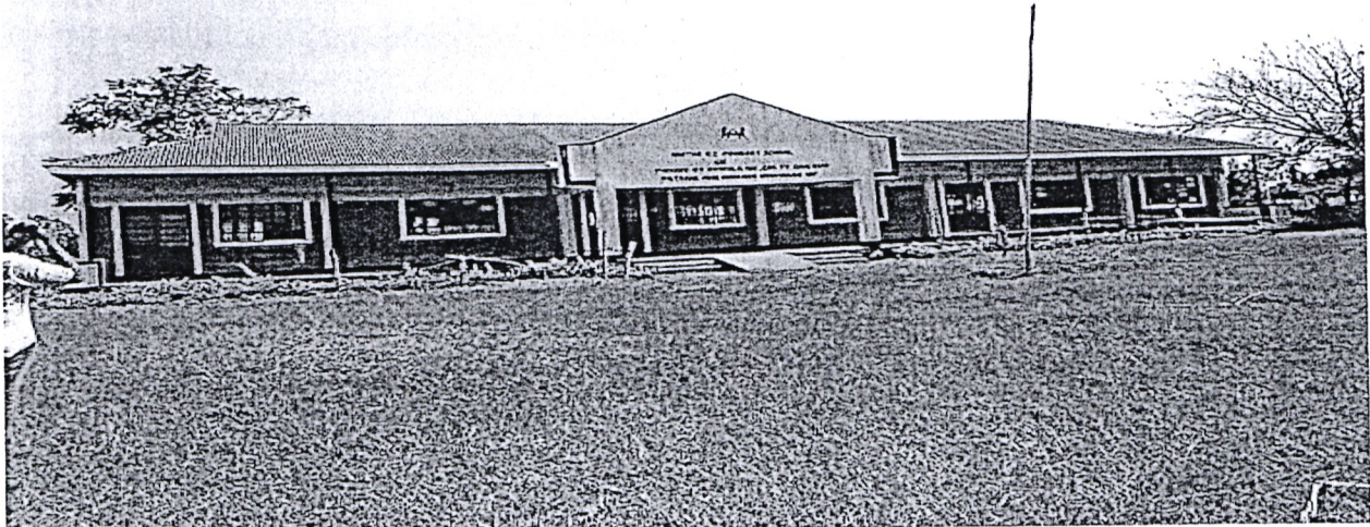
NAMUNINGIE PRIMARY SCHOOL - CONSTRUCTION OF 3 CLASSROOMS FY 2018/19
