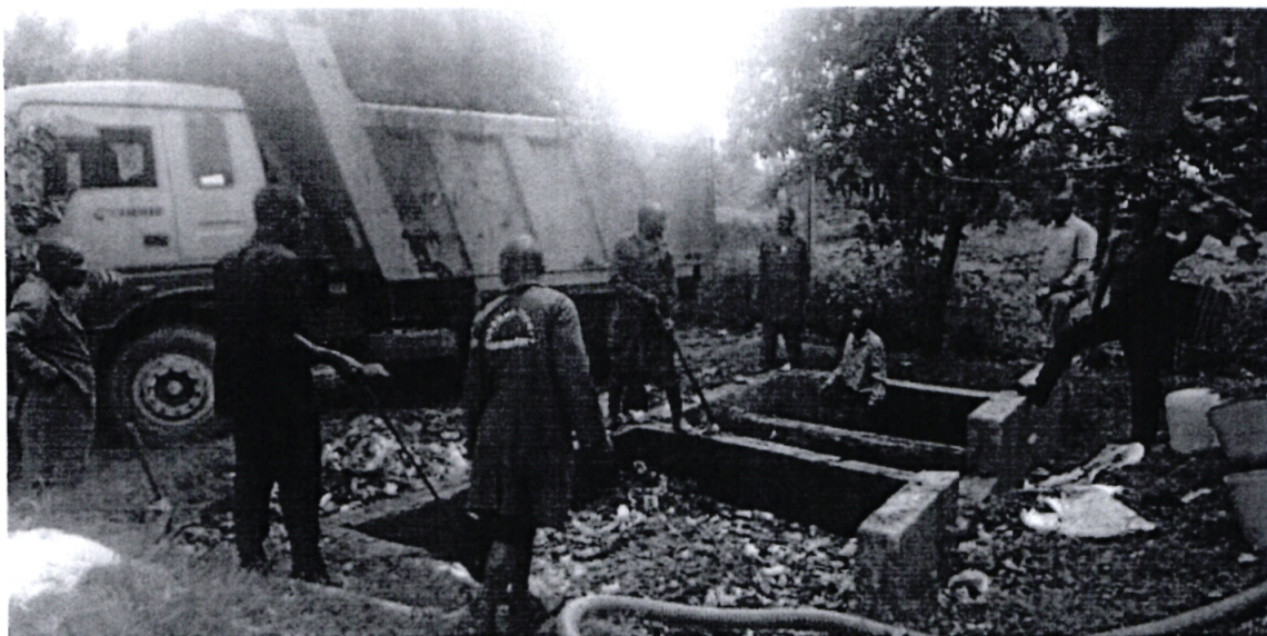
The service provider emptying the composite pit
