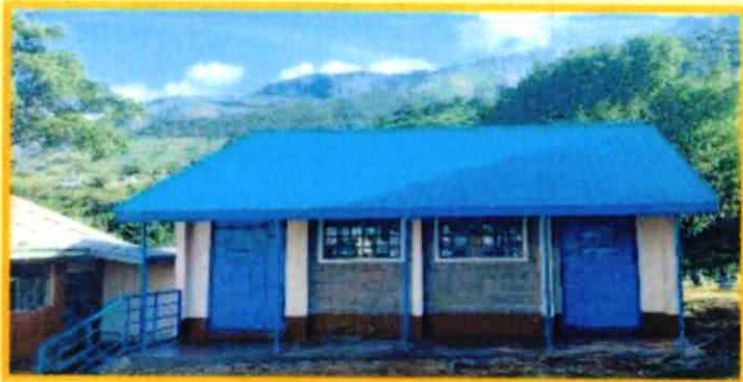
Construction of a classroom at Chepsigot Special School in Elgeyo Marakwet
