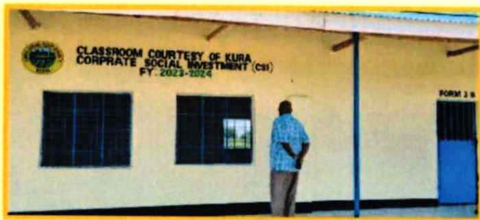
Construction of a classroom at Hudhile Primary School in Wajir County
