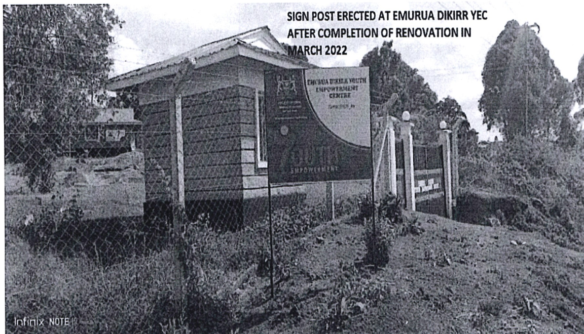
Photo 2: Emurua Dikirr Youth Empowerment Centre (YEC) after undergoing renovations
