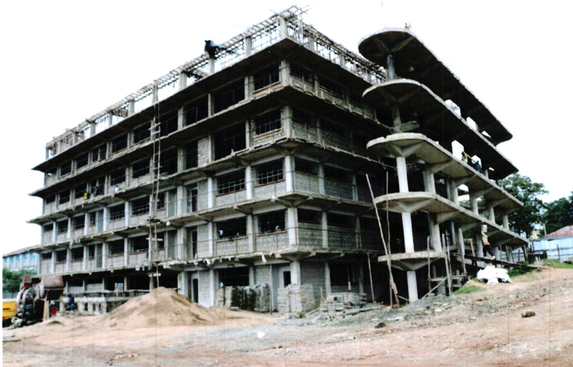
Fig 2. Tuition Block under construction
