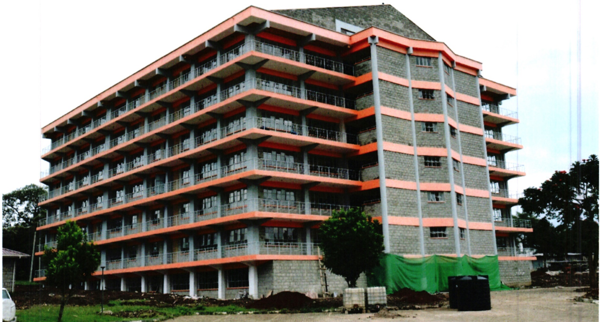
Fig 1: The Office Block under construction
