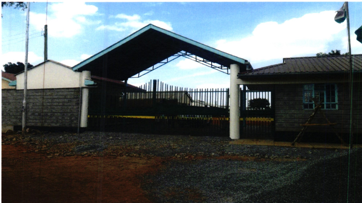
Completed Kamae Borstal Institution Main Gate
