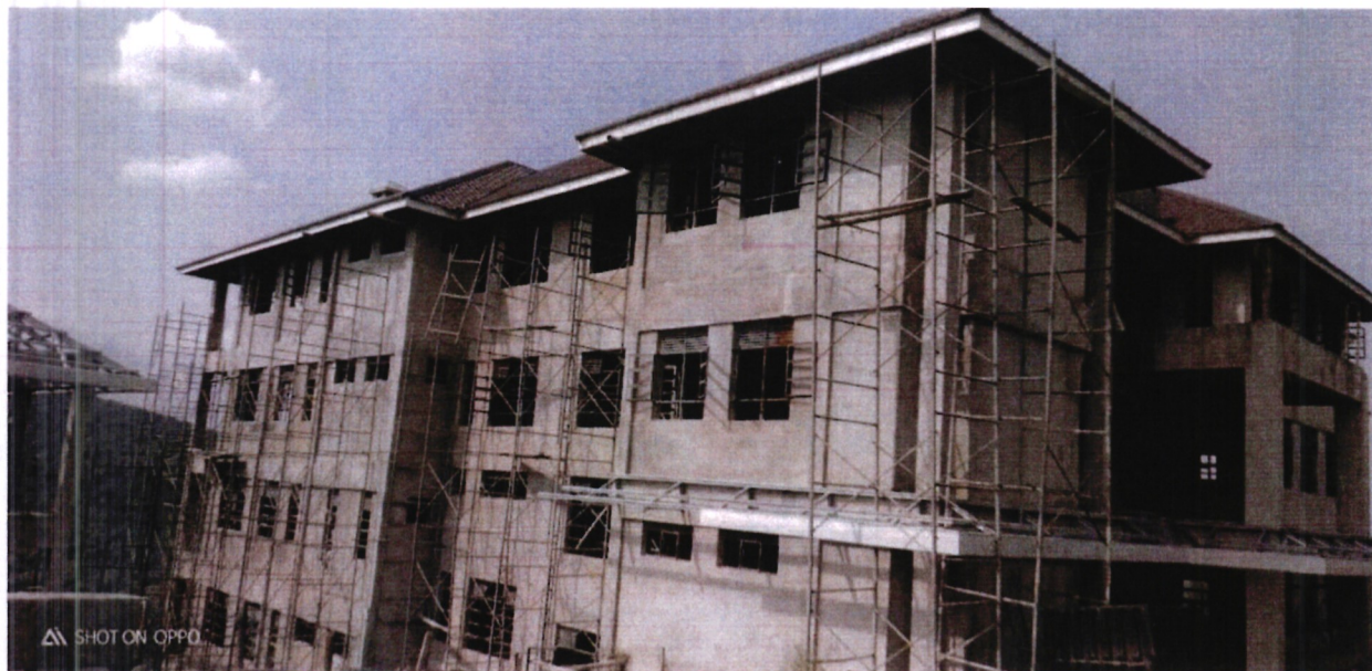
Photo 3. Work in progress at CWSK Murang'a Foster Care (Floor Elevation)
