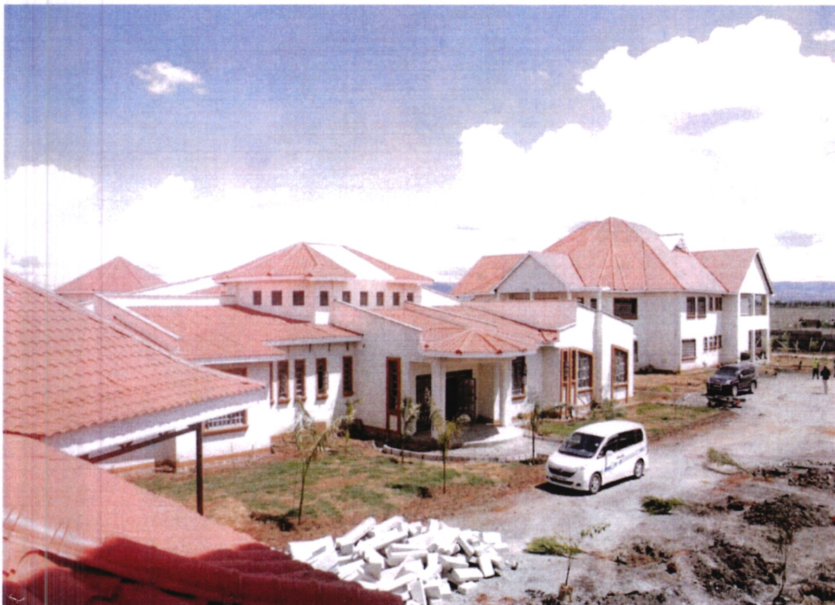
Photo 1. A section of Joska project (front elevation maisonettes and bungalow)
