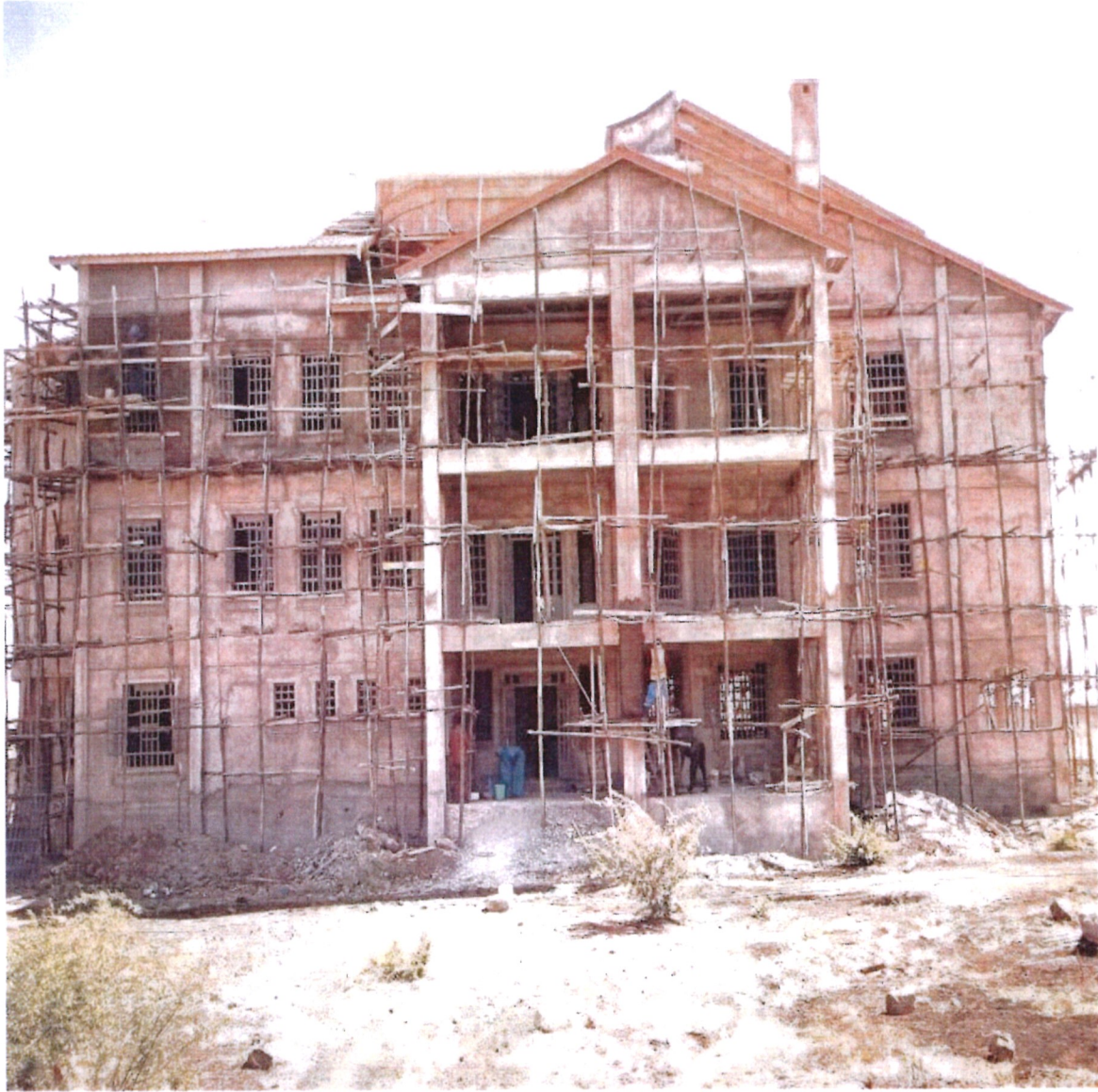
CWSK Isiolo: Foster house 3 in progress
