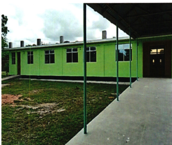
Newly operationalized Samburu Hospital Theatre
