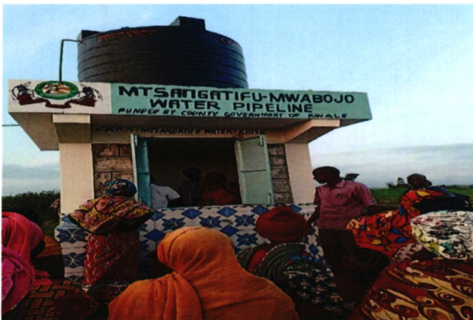
Mtsangatifu-Mwabojo Water Pipeline
