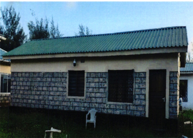
Data Center in Mvindeneni
