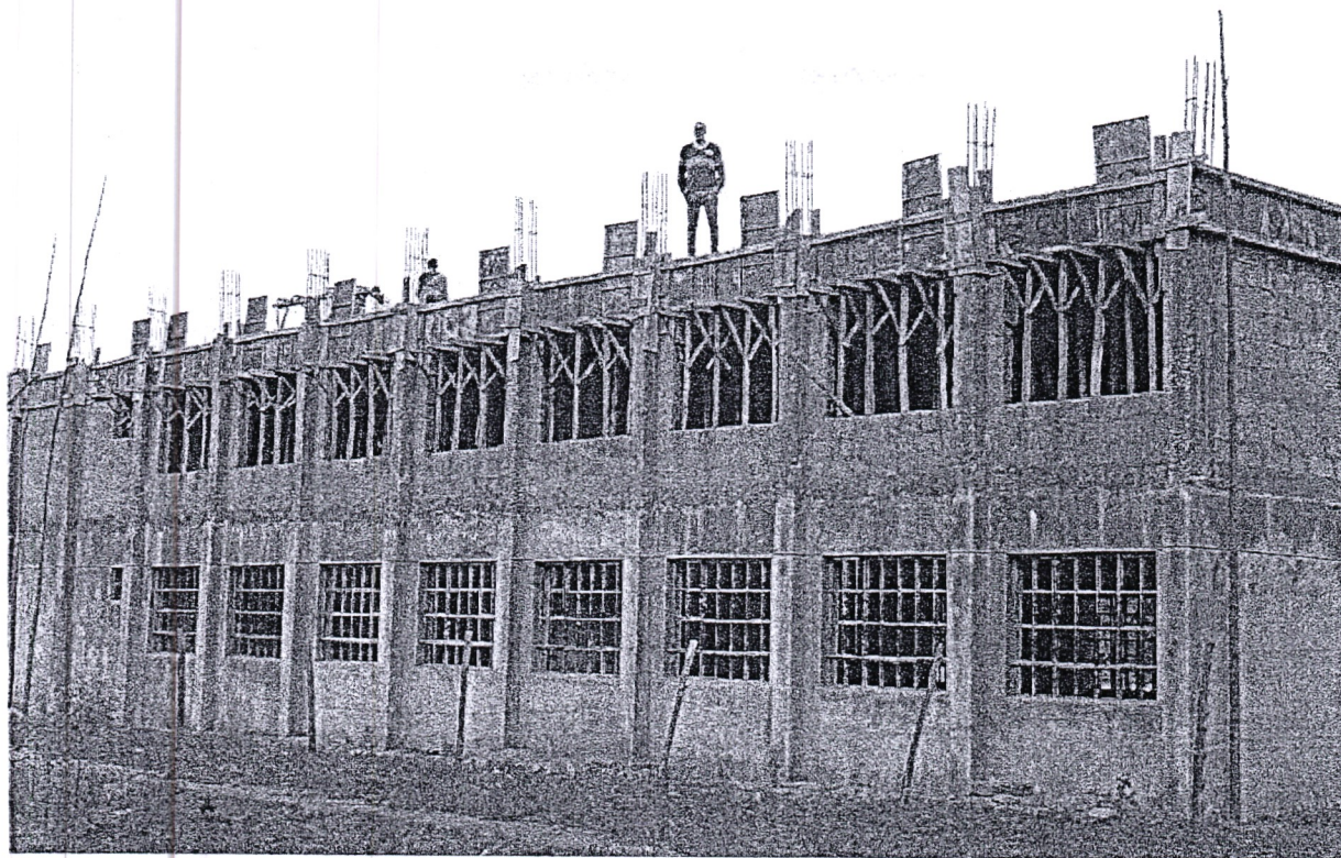
FIG 03. ONGOING CONSTRUCTION OF MATUNGU KMTC
