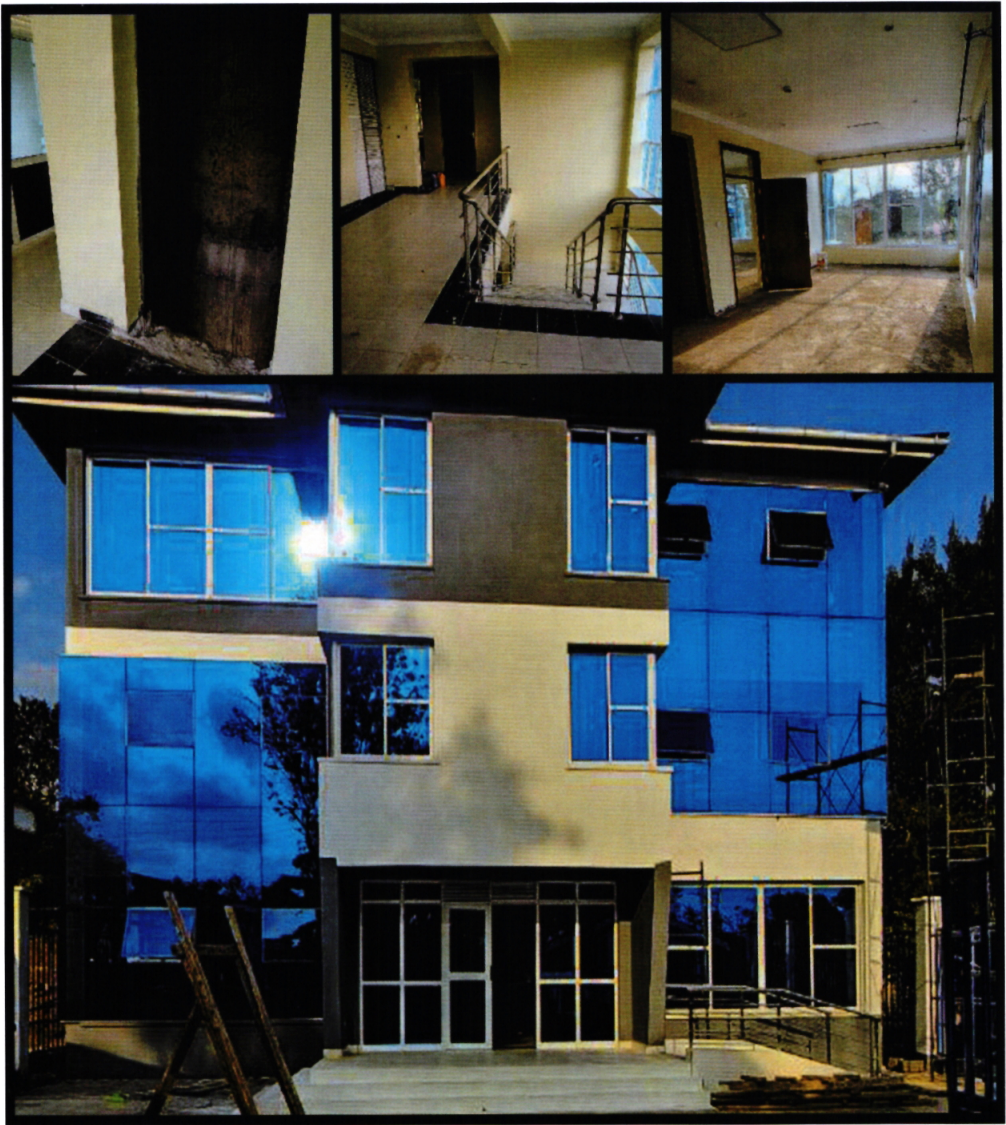
Ongoing construction of TSC Machakos County Office
